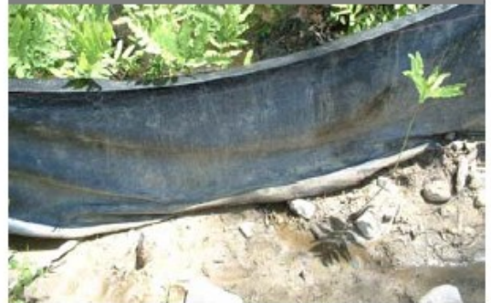
Working Silt Fence with Hay Bale Reinforcement
