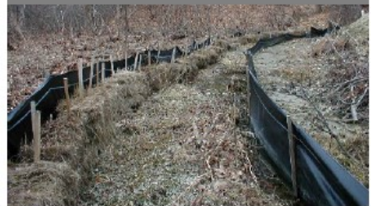
Working Silt Fence with Hay Bale Reinforcement
