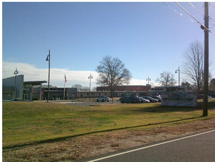
Bolton High School 72 Brandy Street, Bolton, CT
