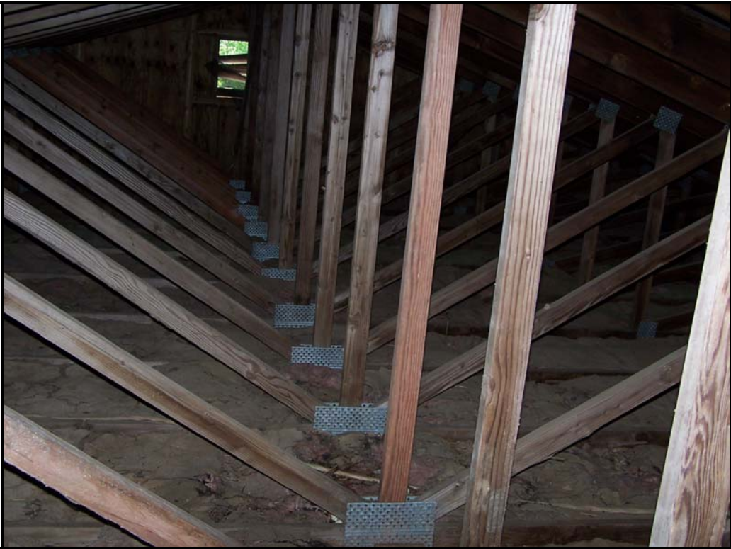
Photo BN1 – Wood roof trusses above the milking barn.
