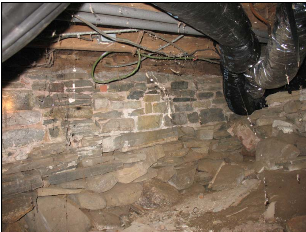
Photo B9 – Addition stone foundation wall with brick capping.
