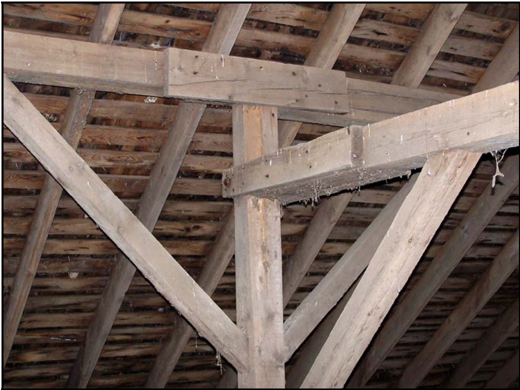
Photo BN9 – Main barn interior cross bay framing with reinforcing pieces.
