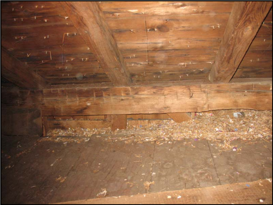
Photo P4 – Main house roof eave girt with rafter connection.
