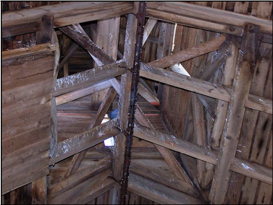
Photo BN6 – Main barn center roof cupola framing.
