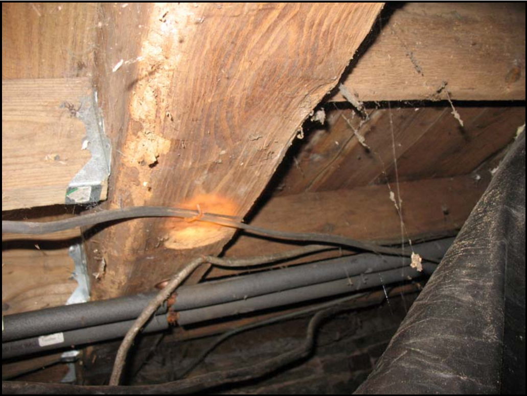
Photo B8 – Addition with original girder and old and new joists.
