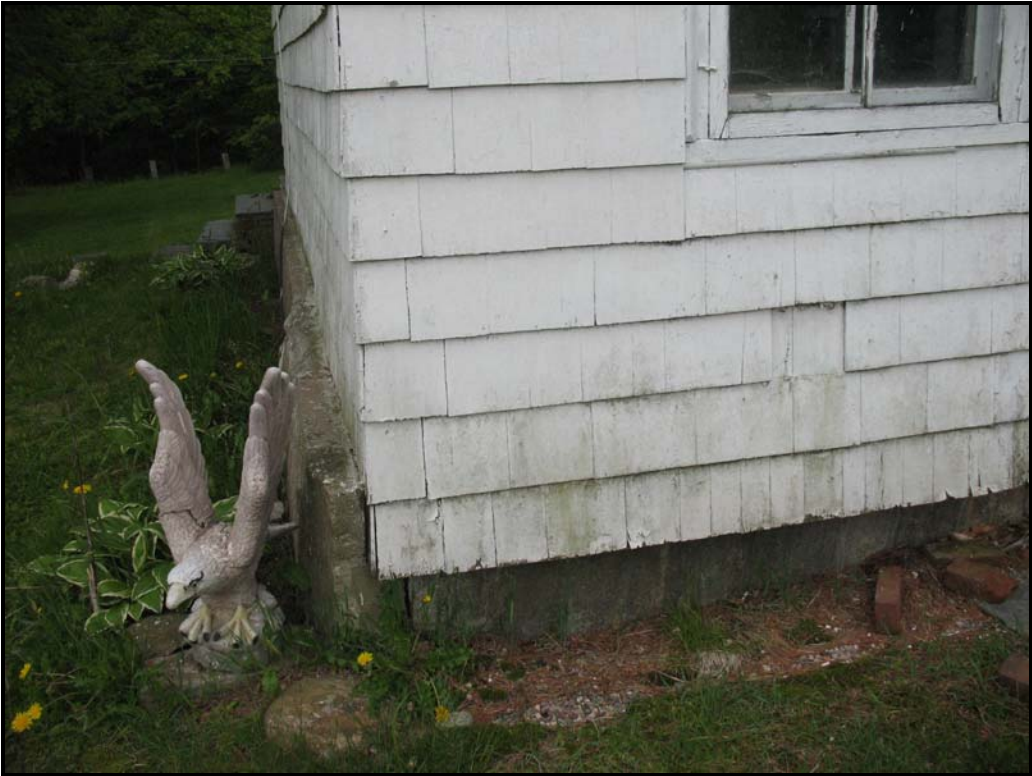
Photo EP5 – Cast-in-Place concrete foundation wall fascia at east side.
