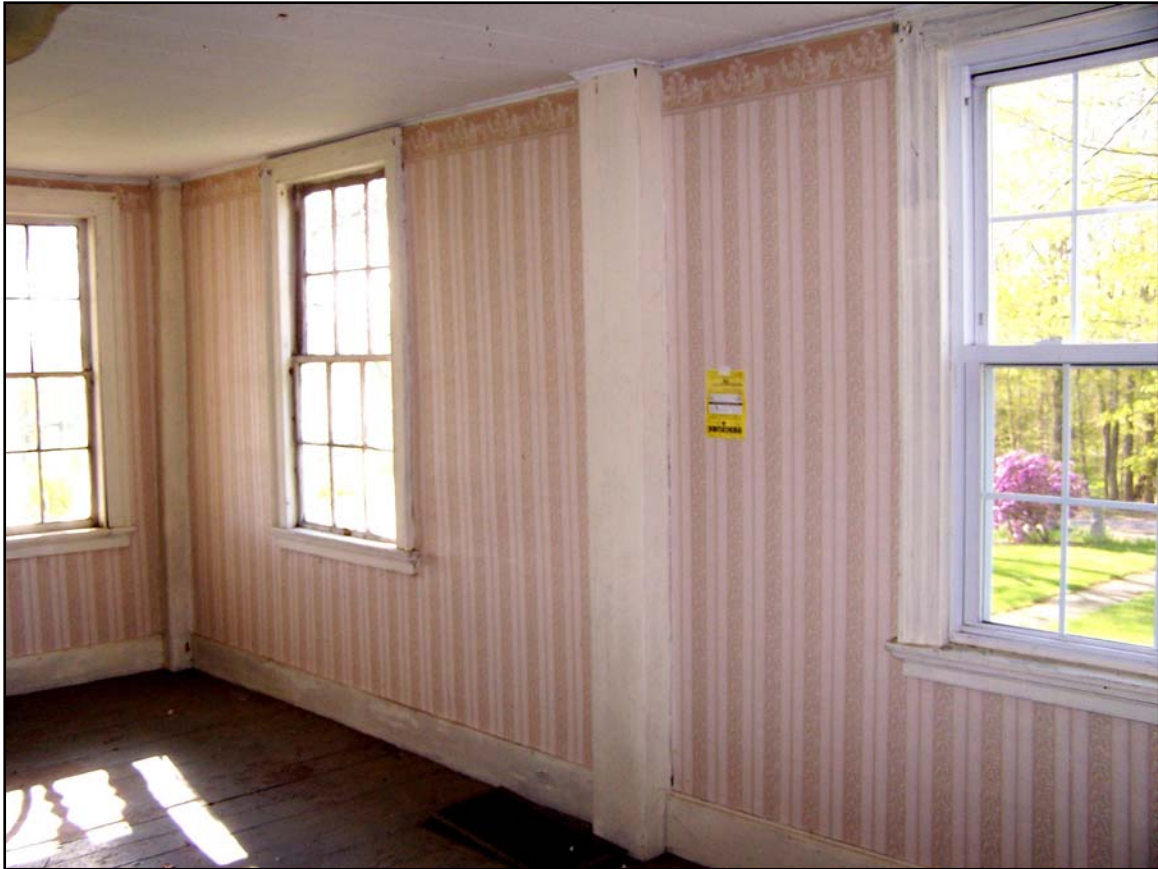
Cased posts in the first-floor front room, camera facing southeast.
