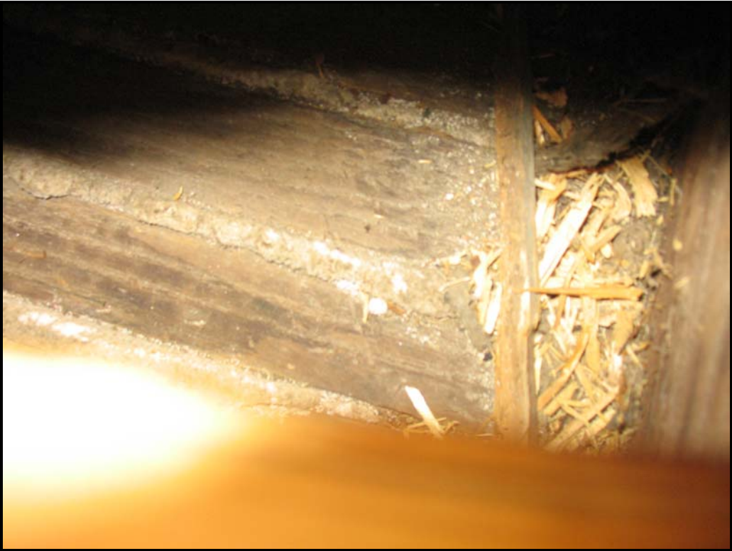
P10 – Addition second floor joist with T & G deck.
