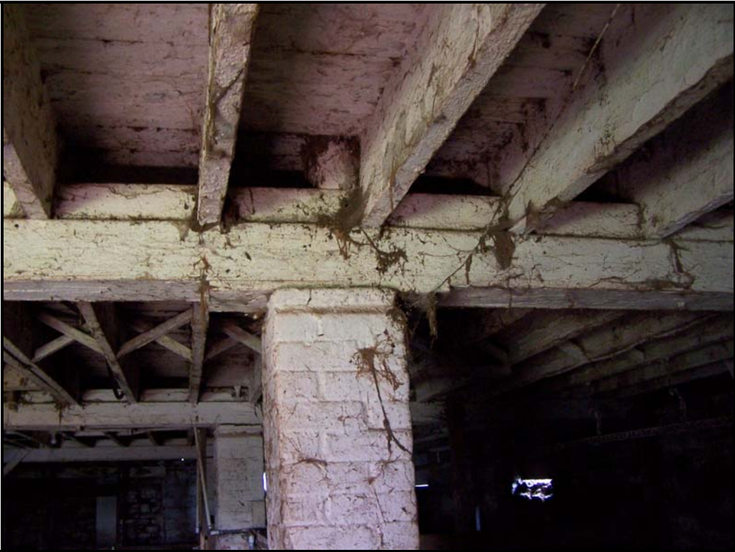
Photo BN13 – Top of main barn basement supporting brick pier.
