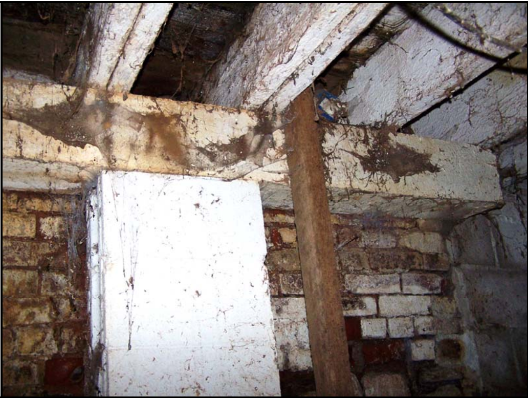
Photo BN16 – Main barn basement end wall with vertical bracing pilaster.
