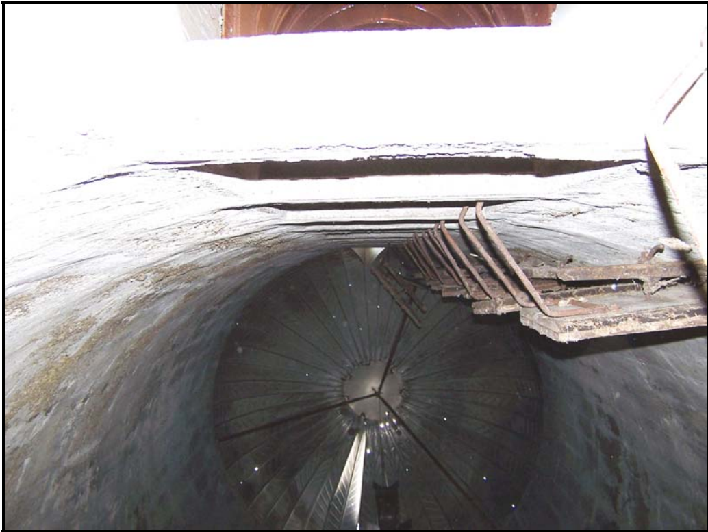
Photo BN20 – View inside concrete block silo looking up towards roof.
