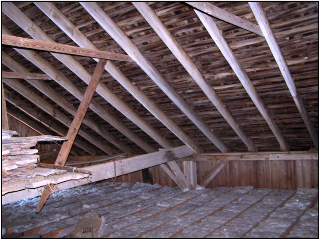
Photo BN10 – Minimal wood roof structure above the south shed building.
