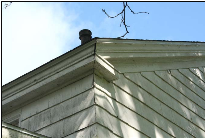
Photograph House-10b: Cornice molding on the kitchen ell.
