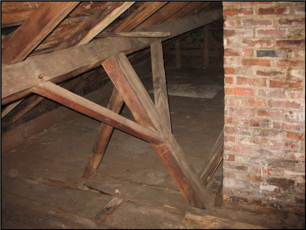
Photo P2 – Main House attic central braced purlin frame.
