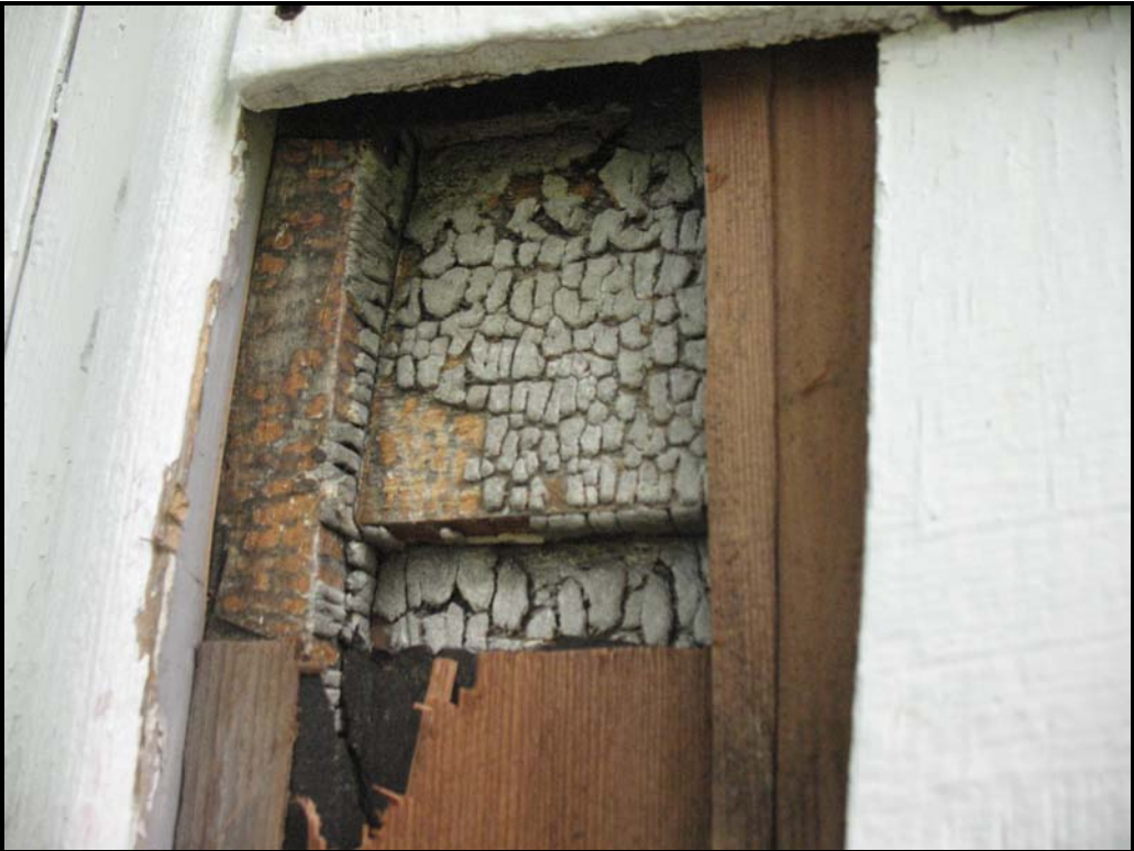
Photo EP2 – Close-up of original clapboard siding.
