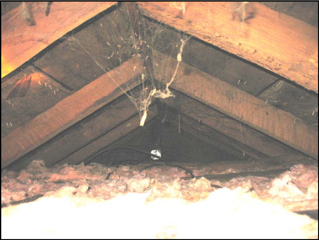
Photo P9 – Addition roof rafters with 1x ridge pole.
