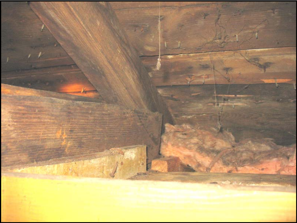
Photo P8 – Addition roof with high collar ties.
