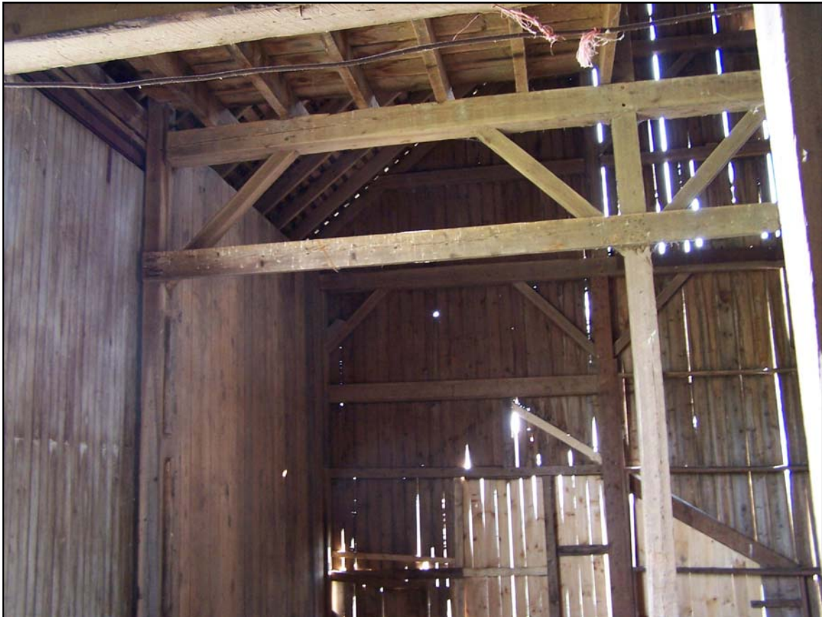
Photograph Barn-4: Interior of barn, showing typical post-and-beam framing.
