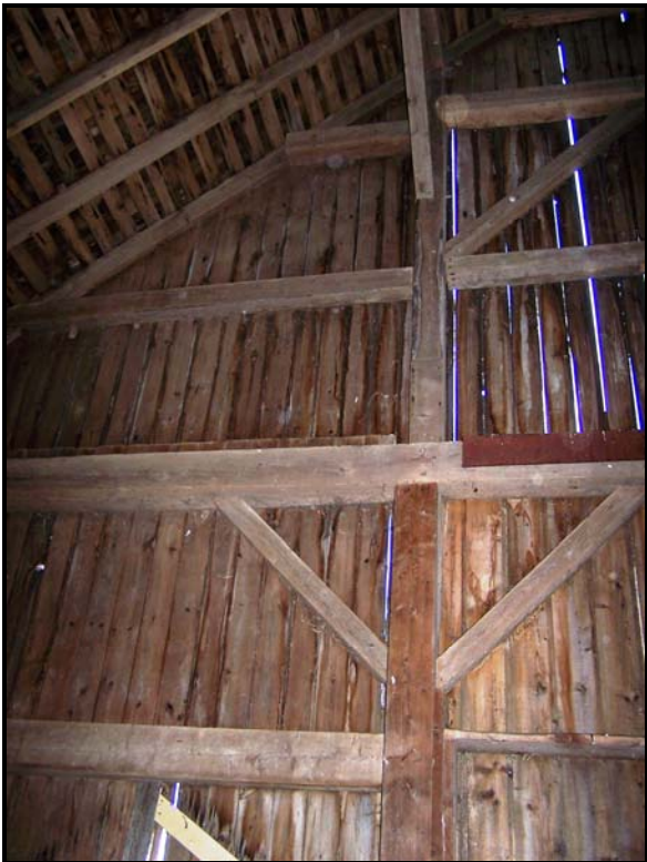
Photo BN3 – Main barn typical end wall framing with airspaces.
