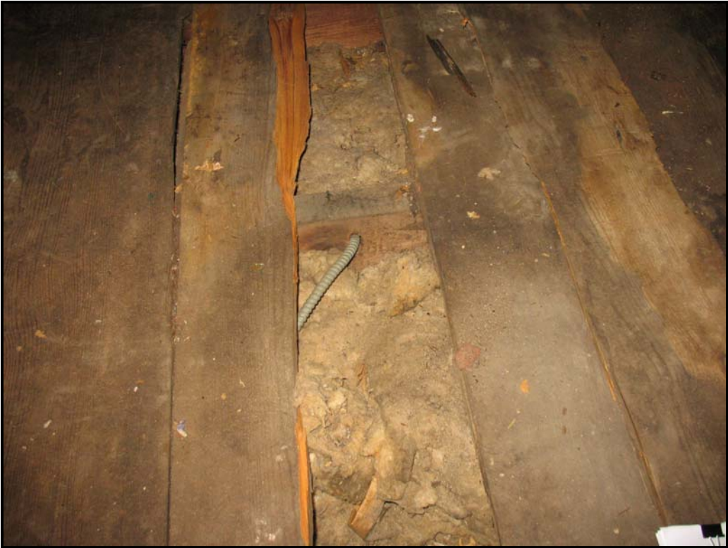
Photo P1 – Attic joist with insulation.
