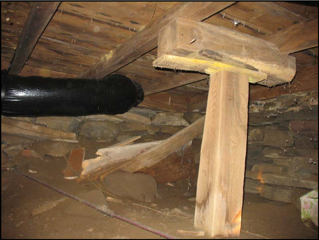
Photo B7 – Addition with first floor old joist shoring system.
