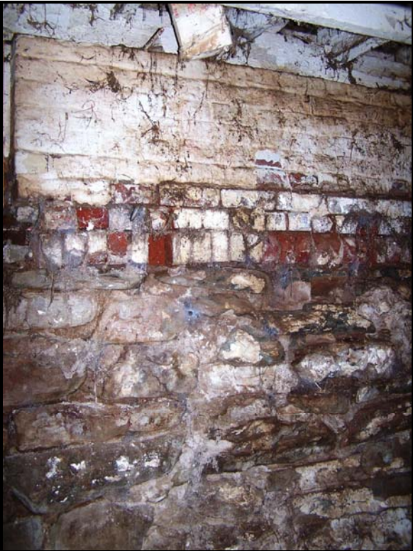
Photo BN15 – Side basement wall construction in main barn.
