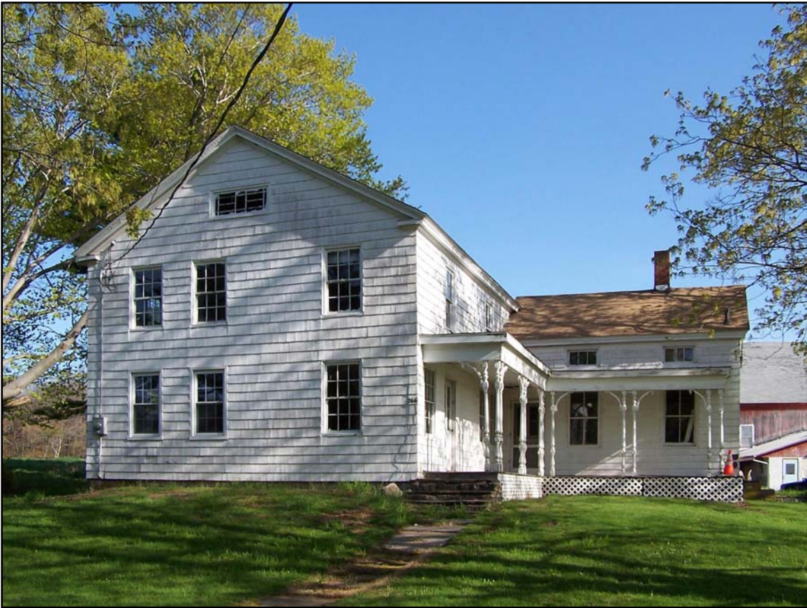
Photograph House-1: Bolton Heritage Farm house, south (front) elevation, camera facing north.
