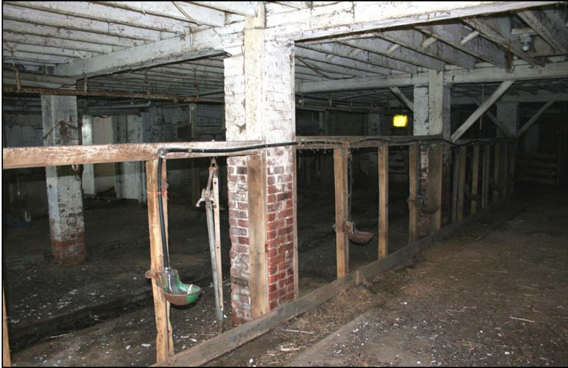
Photograph Barn-7: Interior of barn, lower level, showing added cow stanchions and concrete floor, camera facing southwest.
