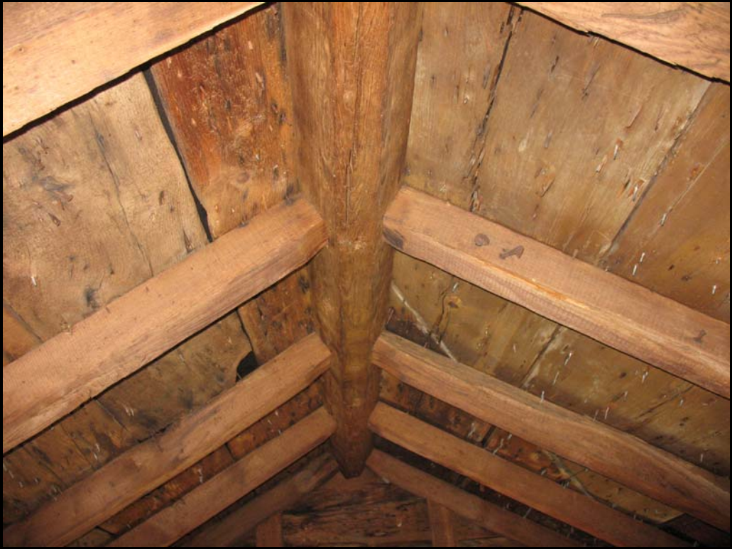
Photo P5 - Main house 5-sided ridge beam and rafter connections.
