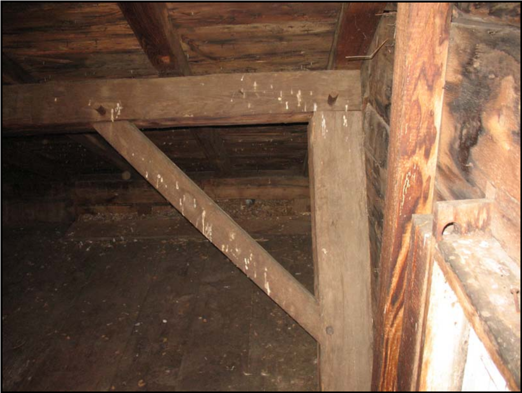
Photo P3 – Main house purlin with end wall column/knee brace.
