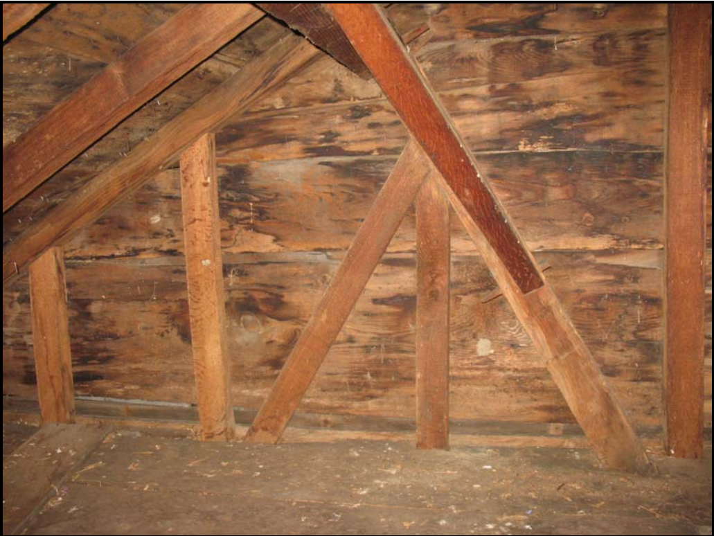
Photo P6 – Main house and end walls with knee braces.
