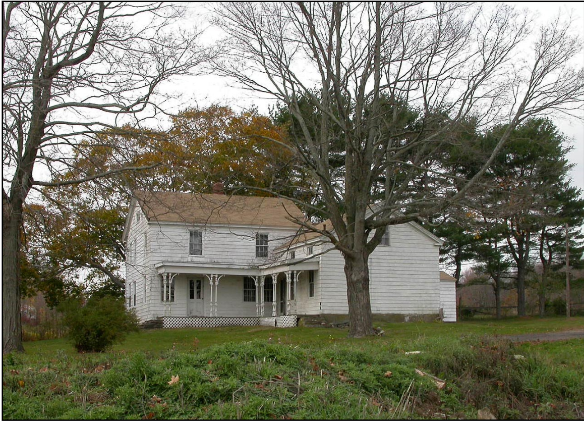
Photograph House-2: Bolton Heritage Farm house, east elevation, camera facing west.
