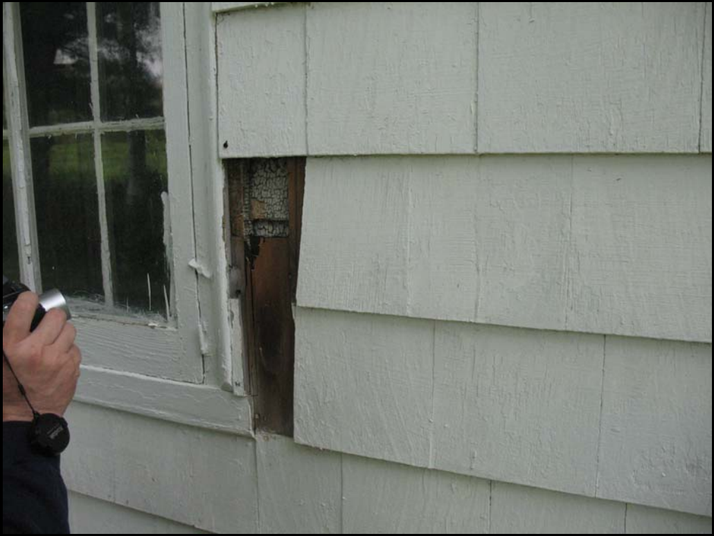
Photo EP1 – Original clapboard painted siding below newer shingles.
