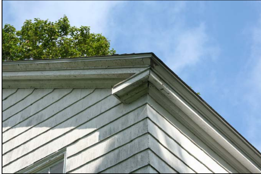
Photograph House-10a: Cornice molding on the main part of the house.
