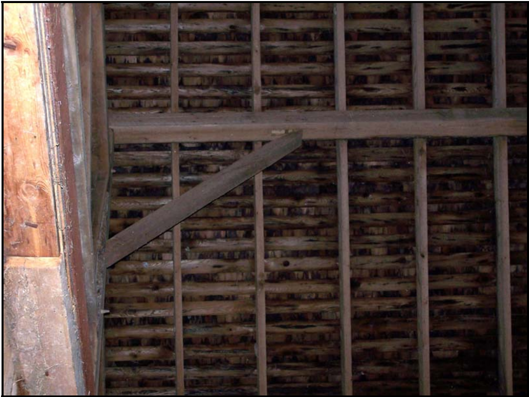
Photo BN4 – Main barn typical roof construction with purlins and rafters.
