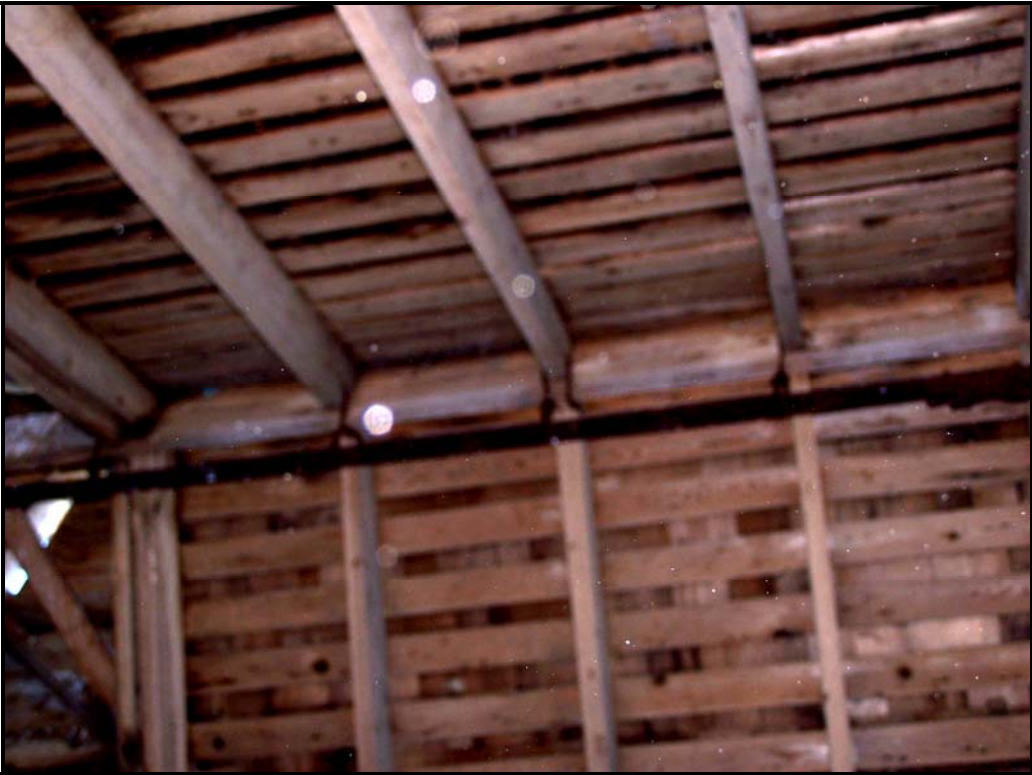
Photo BN7 – Main barn roof rafter/ridge construction.
