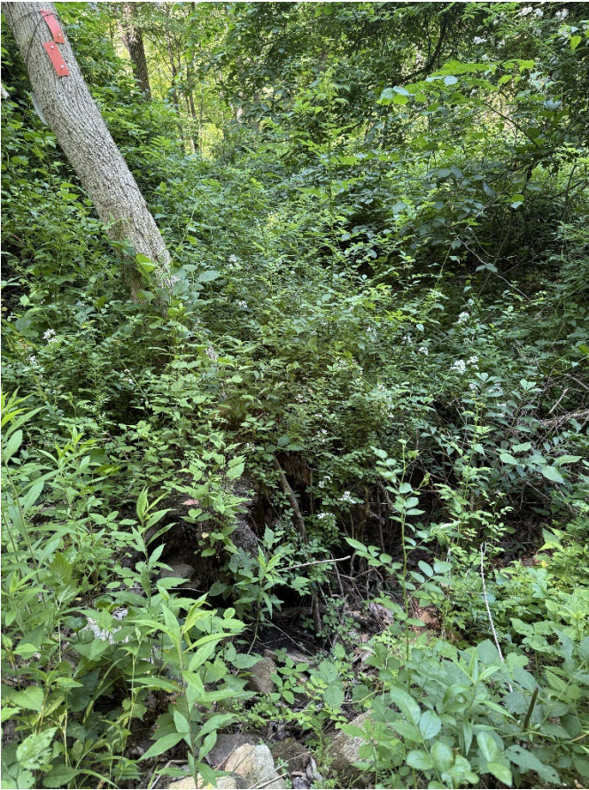
Photos of eroded drainage way to be armored with existing on-site materials
