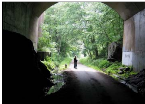
Trail Tunnel at Route 384
