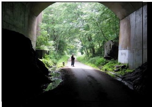
Trail Tunnel at Route 384
