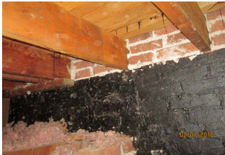
Roof Rafter Pocketed into Exterior Wall
