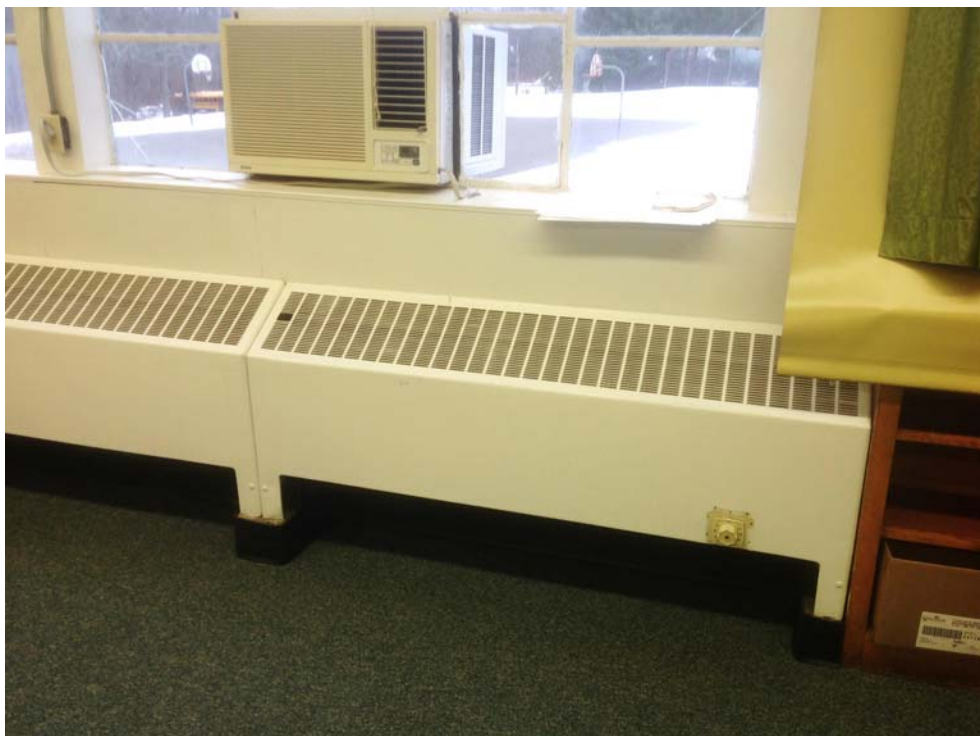
Typical Classroom Radiation
