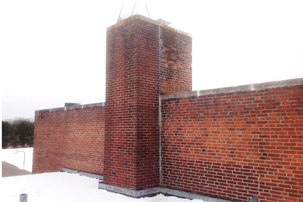
Chimney Stack Looking at Center Section from North Wing Roof
