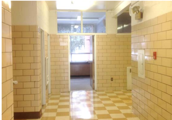
Structural Glazed Tile with Painted CMU Above
