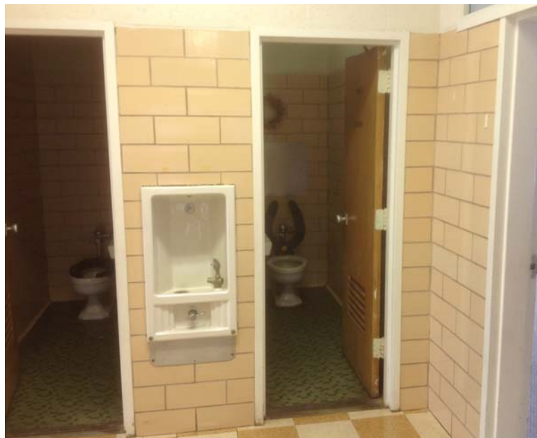
Lower Level Toilet Rooms
