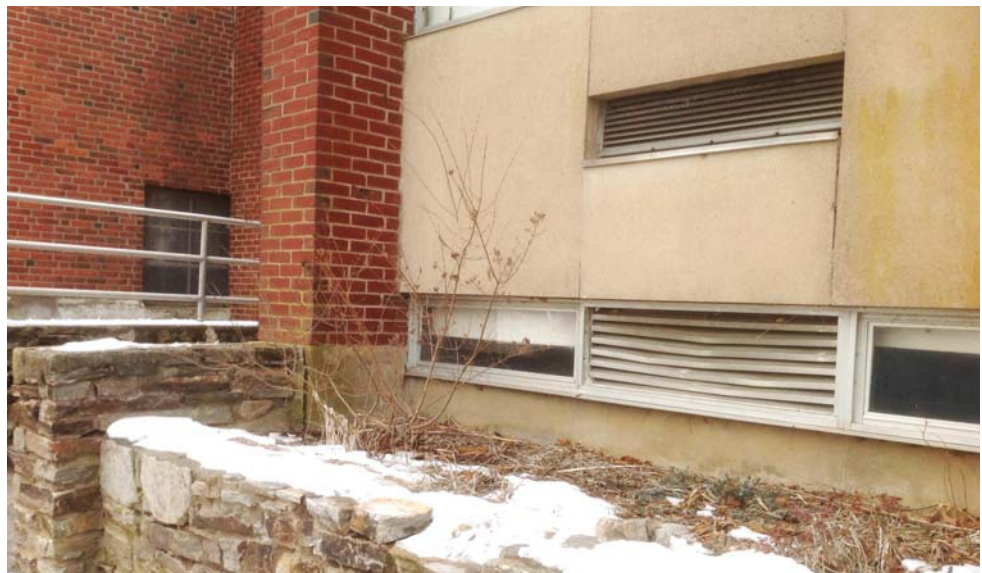
North Wing at East Side - Precast Panels and Louvers
