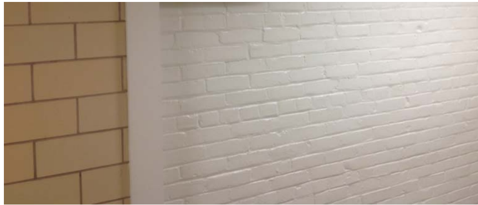
Lower Level Corridor Walls
