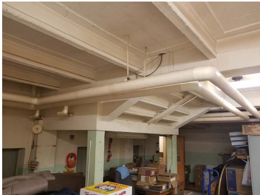
Cast-In-Place and Precast Construction Below Main Entrance
