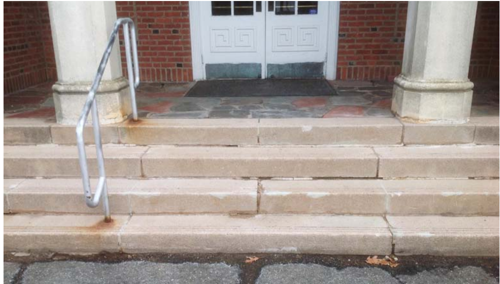
Stairs at Main Entrance
