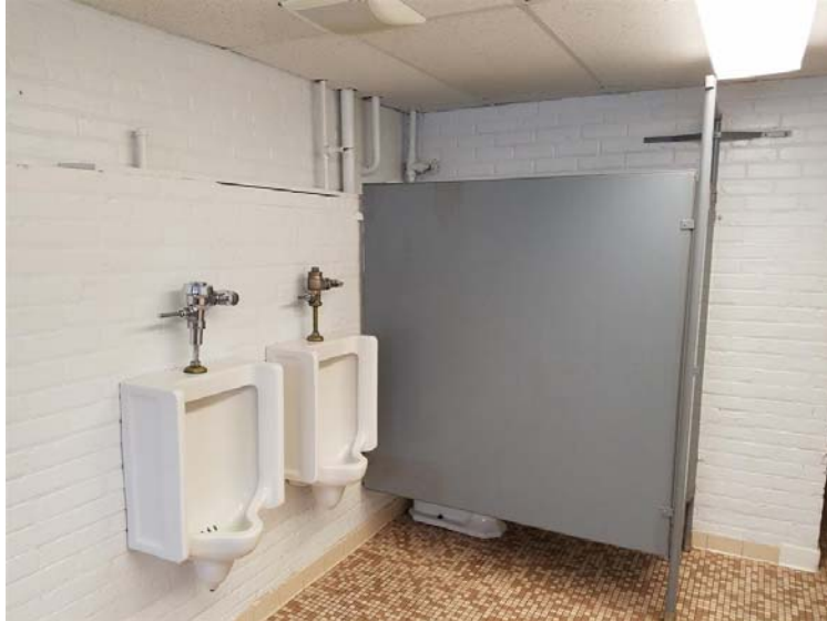
Typical Toilet Room
