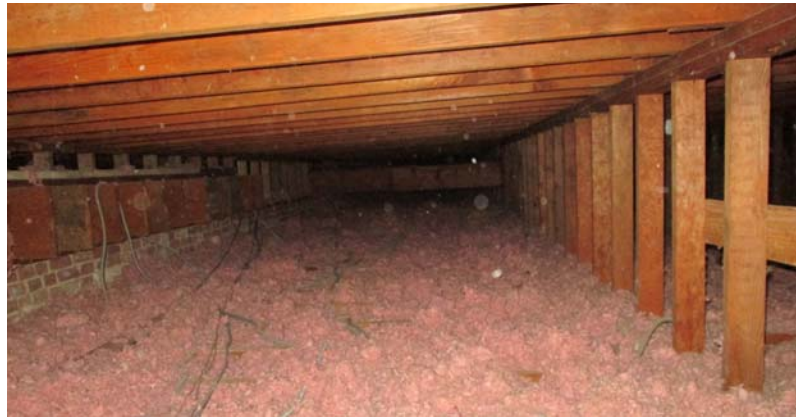
Attic Space Showing Loose Fill Insulation Over Ceiling
