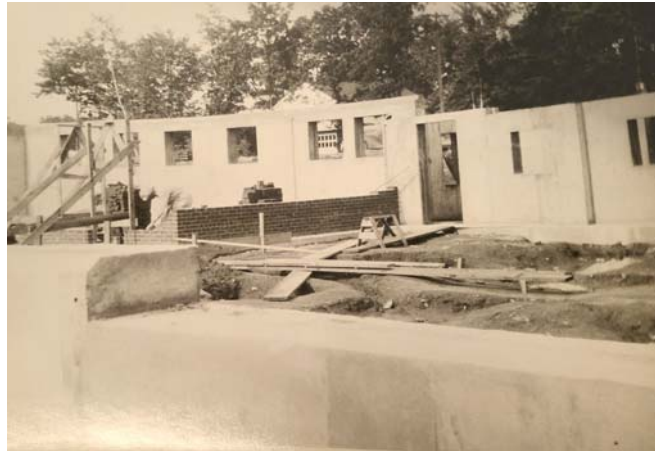
Concrete and Masonry Wall Construction
