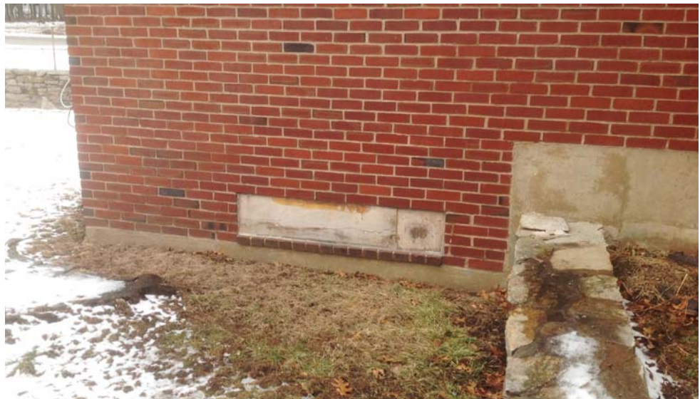
North Wing Lower Level at West Side - Brick and Infill Panel
