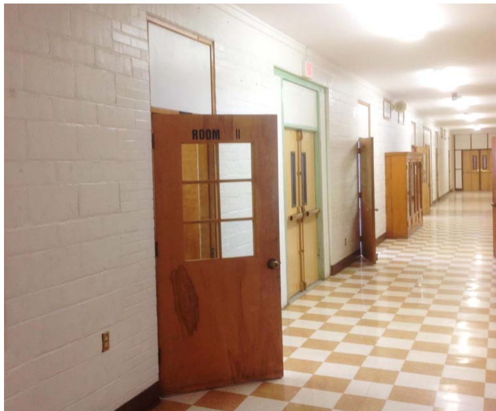
Upper Level Classroom Doors
