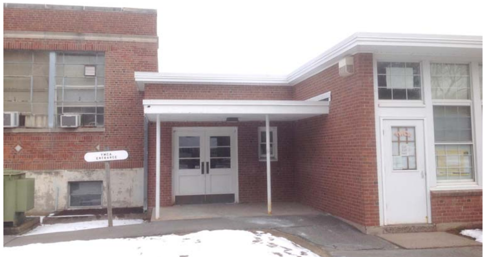
Entrance at South Stair Used for YMCA Daycare
