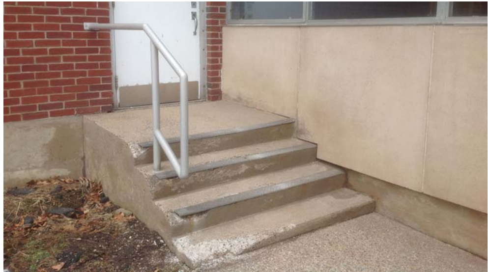
North Wing Upper Level Stair at West Side
