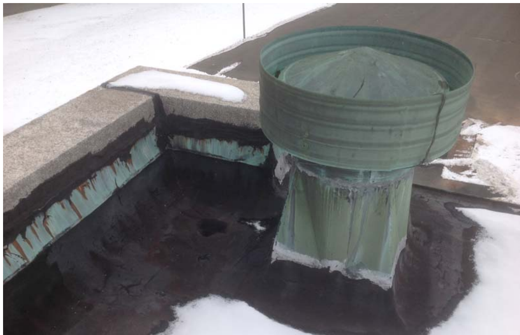
Roof Vent and Parapet
