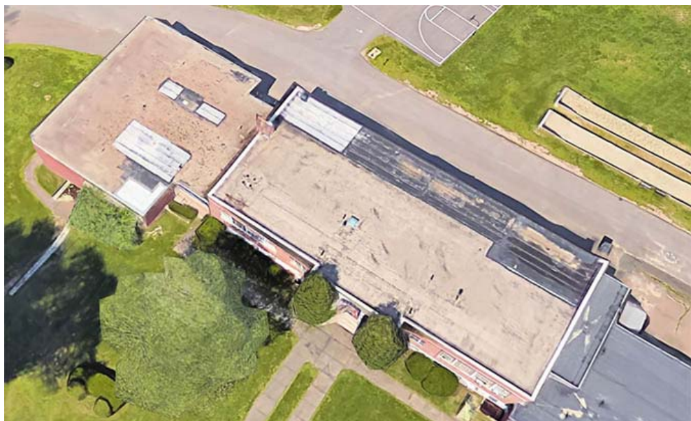
Aerial View of Roof
