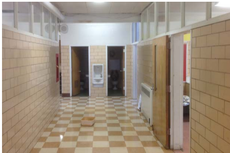
Typical Corridor Flooring
