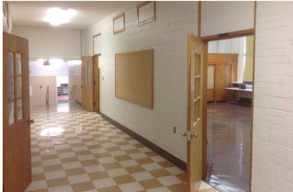
Upper Level Corridor Flooring with View of Classroom Flooring
