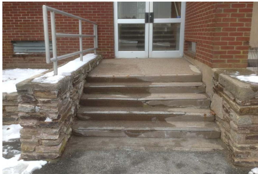
North Wing Lower Level Exit Stair
