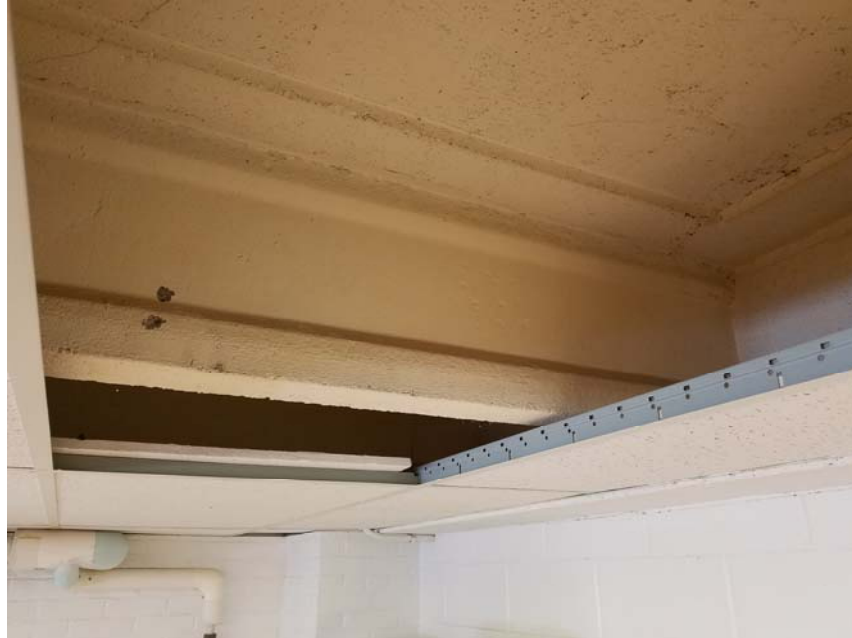
Precast I-Joint with Cast-In Place Slab
