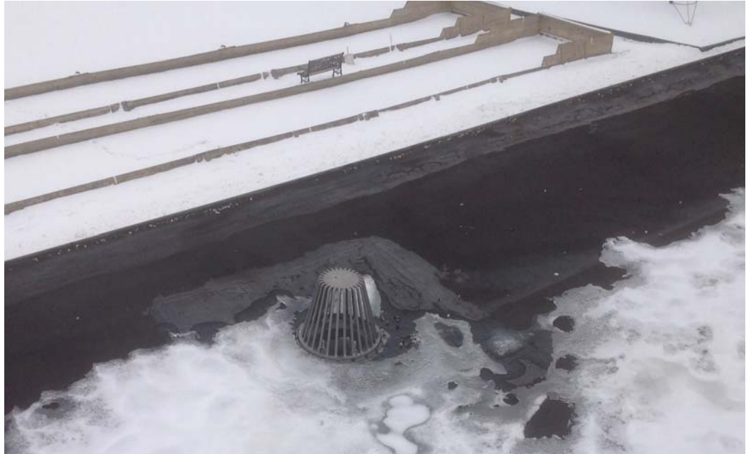
Roof Drain at East Edge
