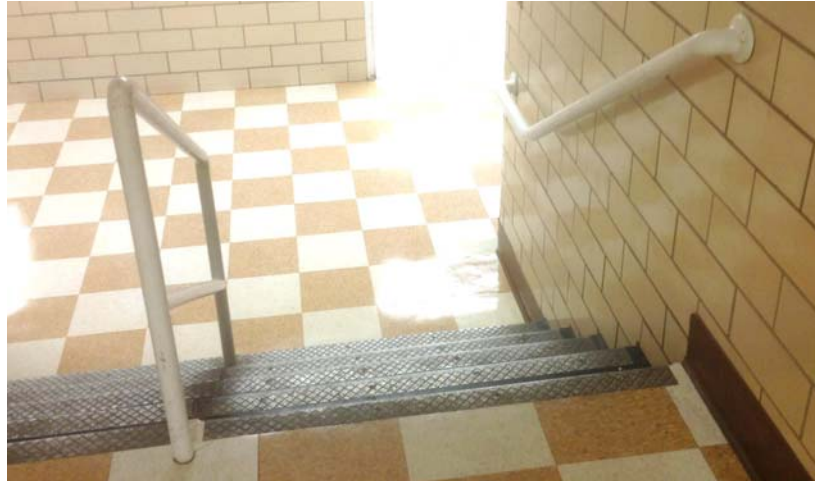
Transition Stair in Upper Corridor from Center Section
