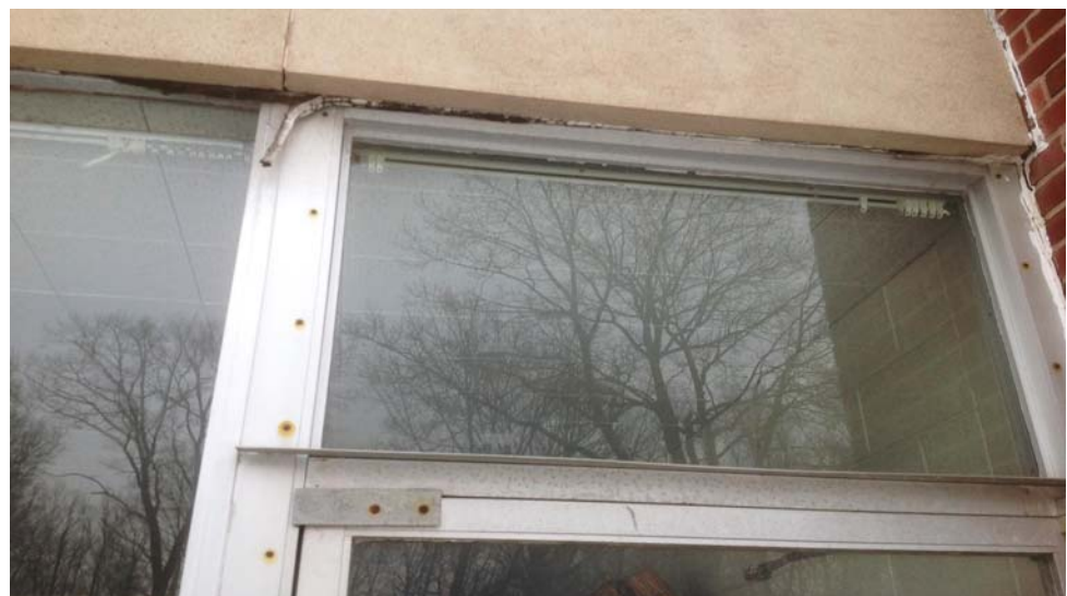
North Wing Curtainwall at Precast Panels
