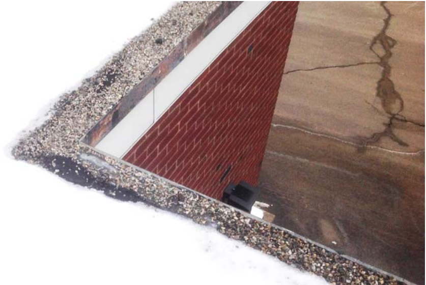
North Wing Roof Edge
