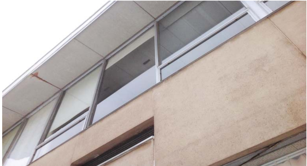
North Wing Curtain Wall
