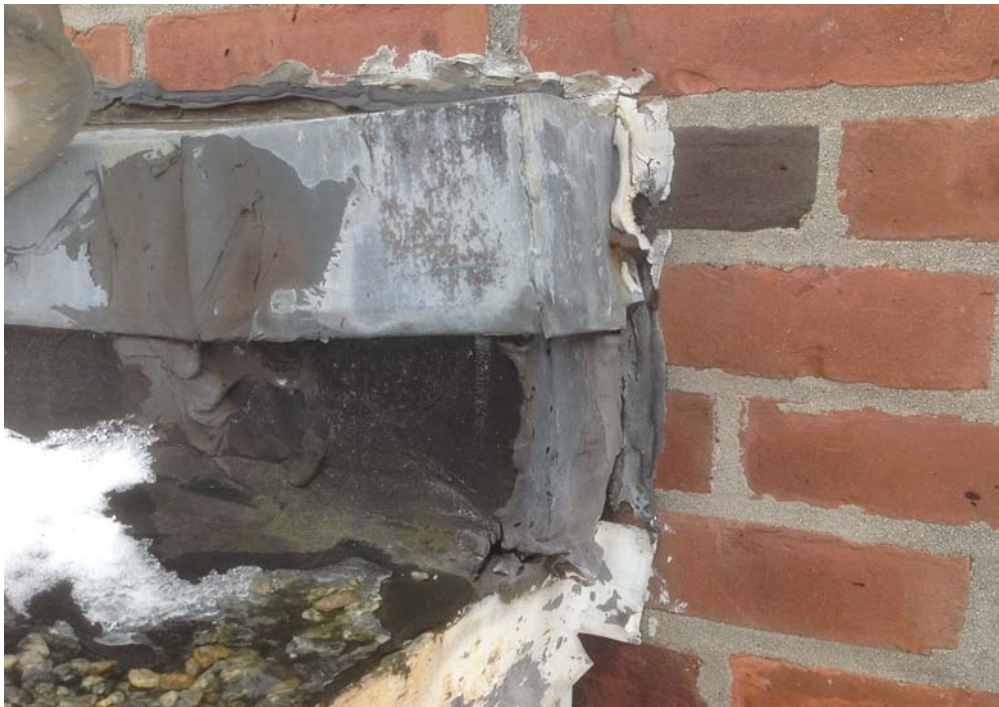
North Wing Roof Joint Against Center Section
