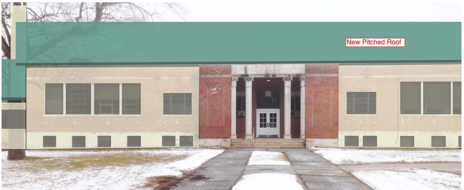
Partial Elevation Showing Pitched Roof
