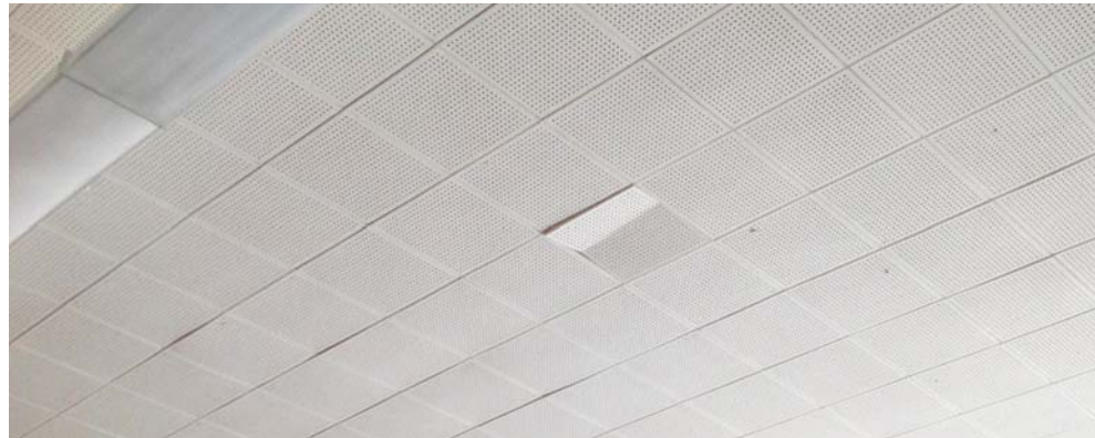
Typical Classroom Fiber-Cane Ceiling Tiles
