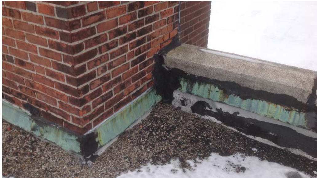
Roof and Parapet at Chimney Stack
