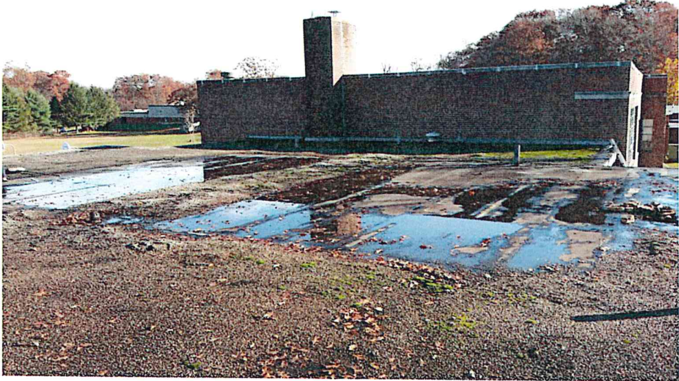
Existing Roof - North Building Roof
