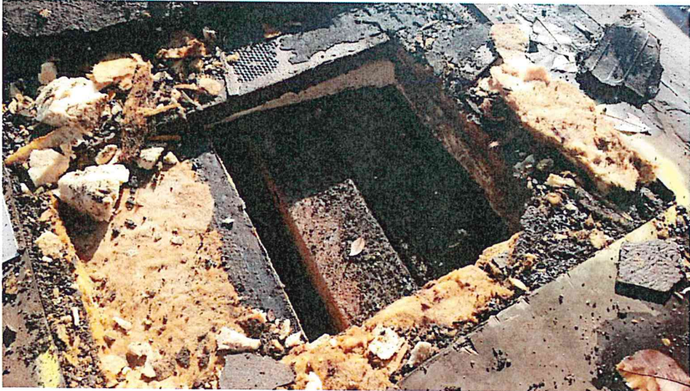
Exposed Roof Deck
