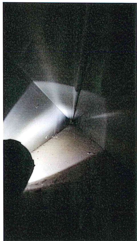
Inside Existing Roof Deck No Water Infiltration Observed
