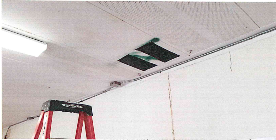
Interior Deck Access Openings
