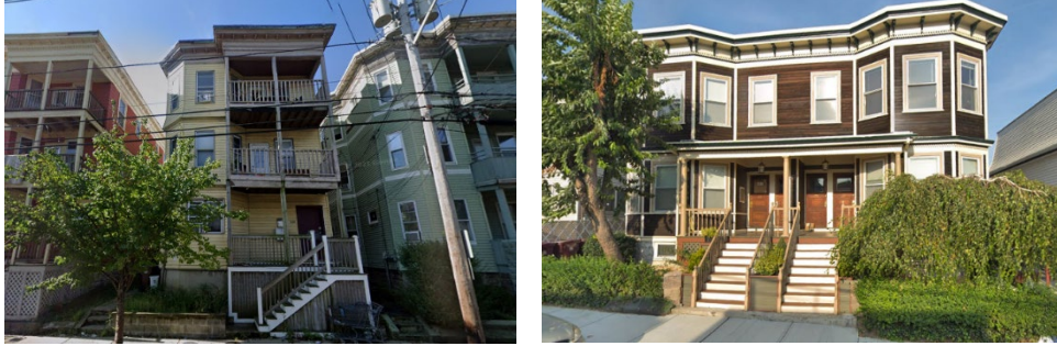
Historic missing middle multifamily housing in Revere. Source: Google Maps.
