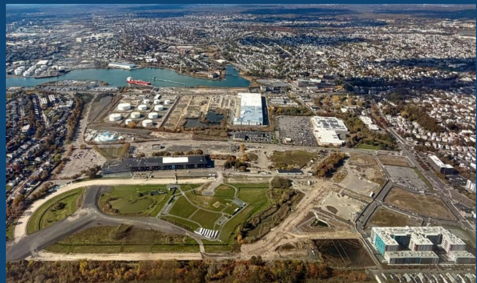
Phase 1R Roadways, R7 Public Parking Lot & Traffic Improvements
