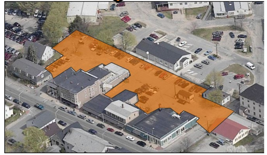
West Concord helped facilitate the sharing of private lots to create a single shared facility, increasing supply for everyone
