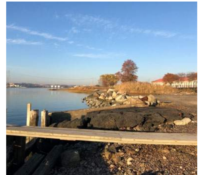
BELOW Existing Boatworks Pier
