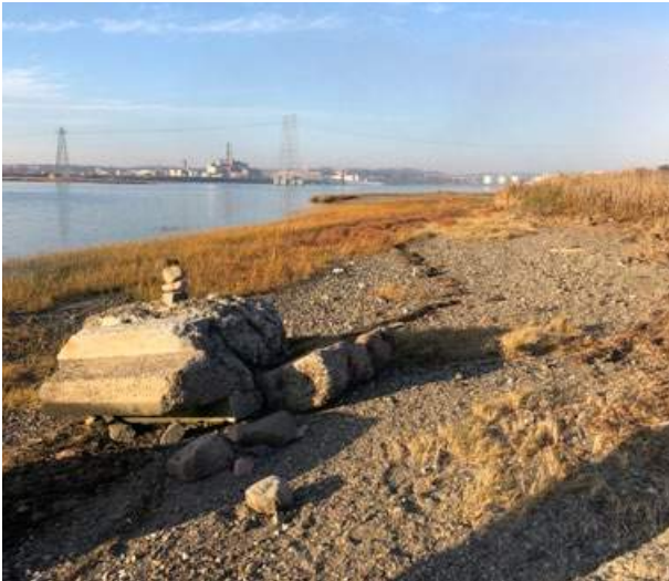
ABOVE Existing Outfall
