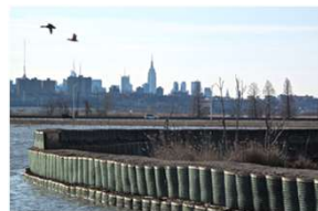
Hesco Barriers, Kane Berm, Hackensack, NJ
