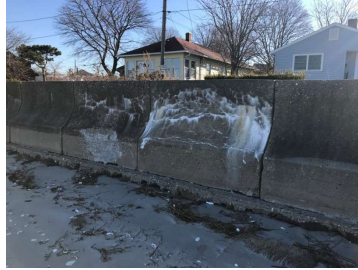
Seawall deterioration
