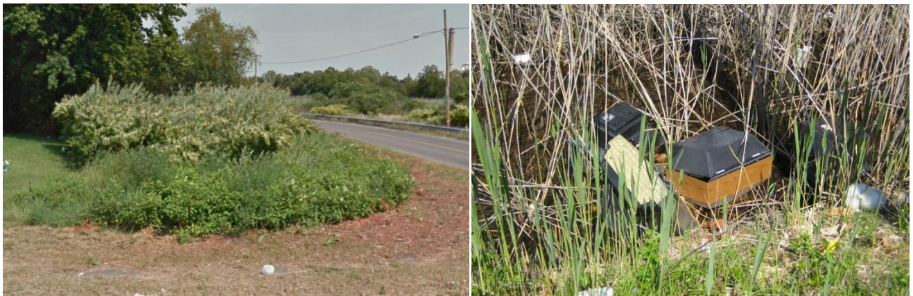
Fig. 2.12 Eastern Ave. Drainage Ditch – South Segment – Left: Overgrown with invasive vegetation; looking north from Bristow Street; Right: Items dumped in ditch. (Photo credit Woods Hole Group, Inc., Appendix 1)
