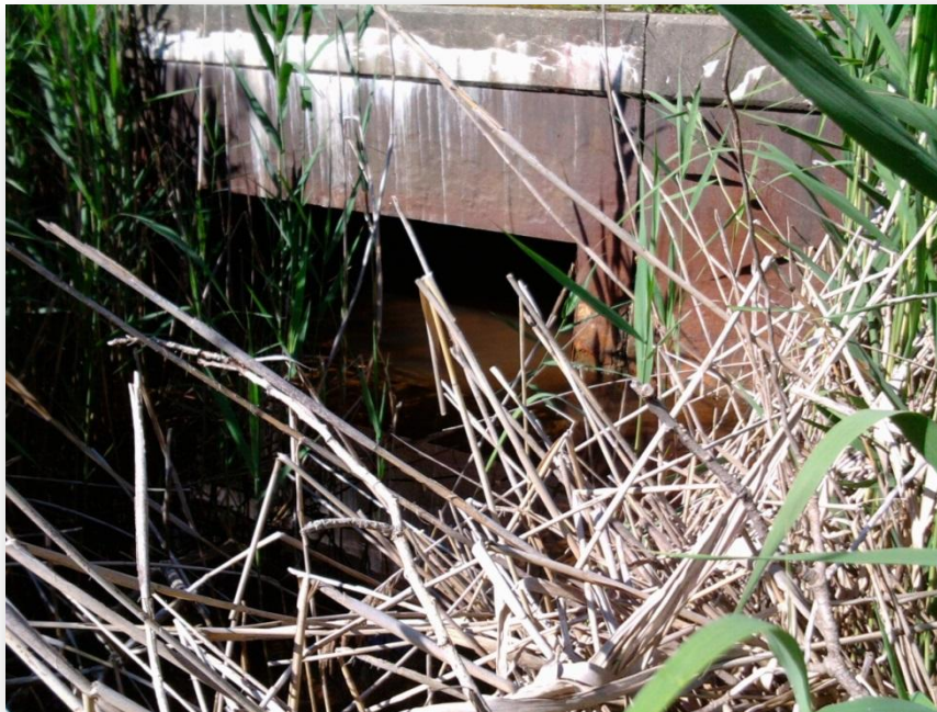
Figure 2-13. Northern end of Pines Creek culvert (culvert A).
