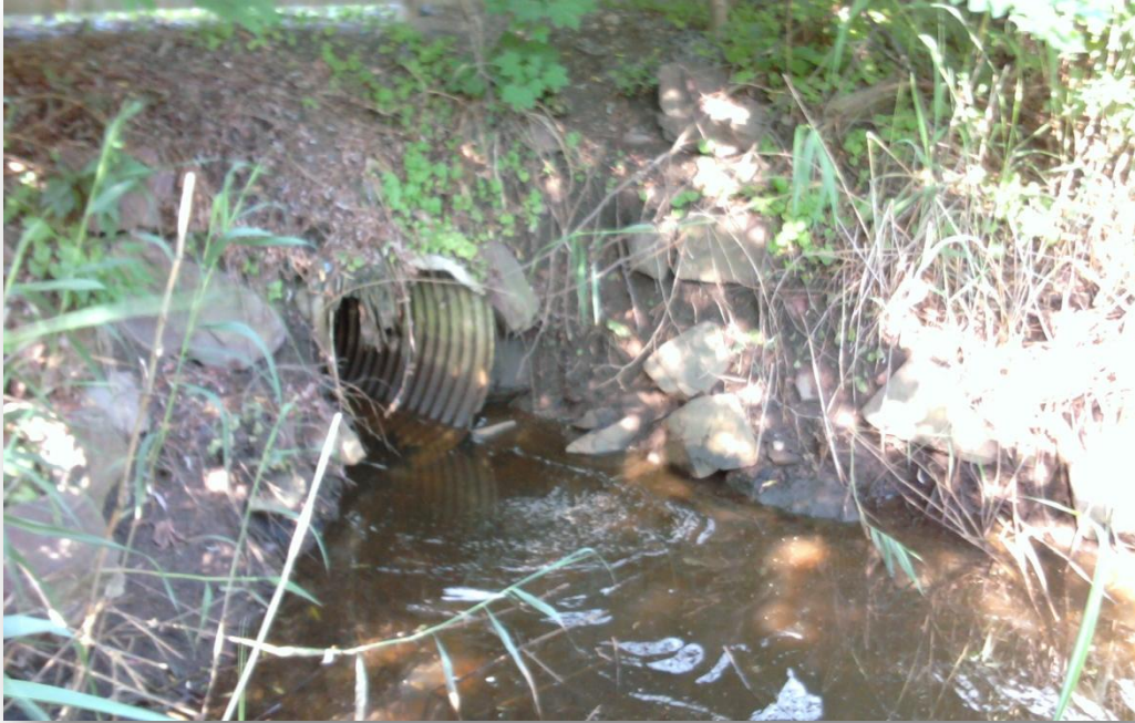
Figure 2-11. Downstream end of parallel culvert (culvert C).
