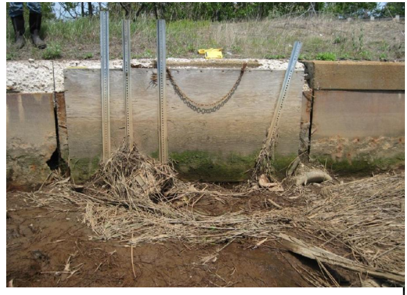
Fig. 4.11 Enlarged View of board on North End of Bristow Street Culvert
