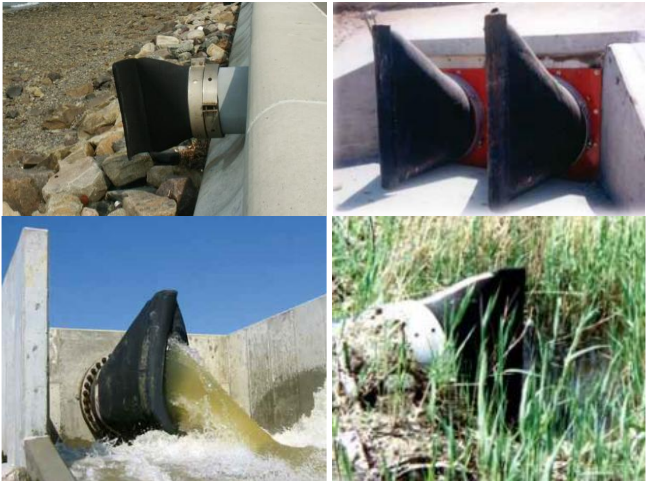
Fig. 4.07 Photographs of Typical duckbill Tide Valves
