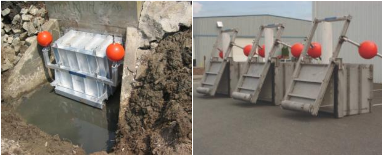
Fig. 4.06 Photographs of Typical SRT, installed (at left) and prior to installation (right)
