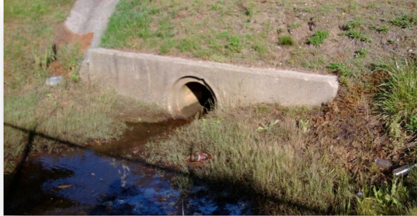
Figure 2-10. Downstream end of small Eastern Avenue culvert (Culvert F).
