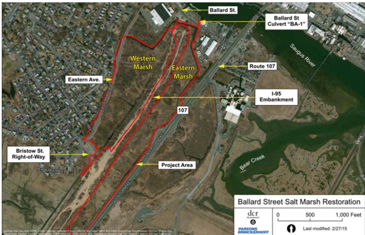
Figure 1. Aerial photograph illustrating main features surrounding the Ballard Street restoration site (source: Modified from Woods Hole Group, Inc.).
