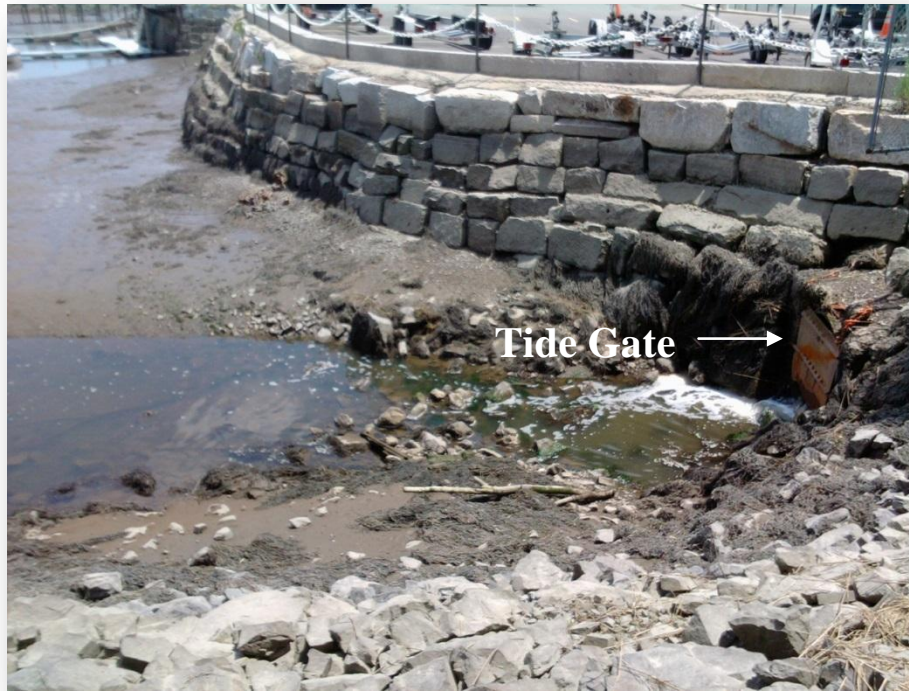
Figure 2-6. Downstream end of Ballard Street culvert with tide gate (culvert G).
