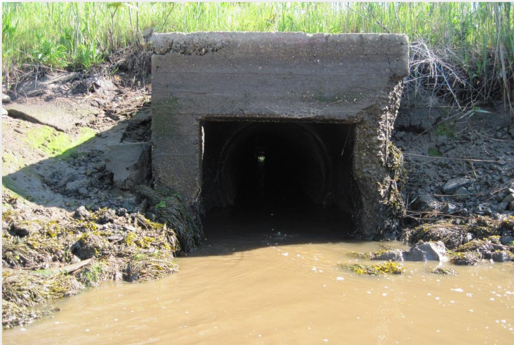
Figure 2-6. Downstream end of Ballard Street culvert with tide gate (culvert G).
