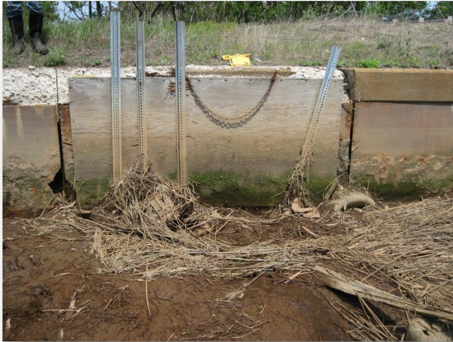
Figure 2-12. Southern end of Pines Creek culvert (culvert A).
