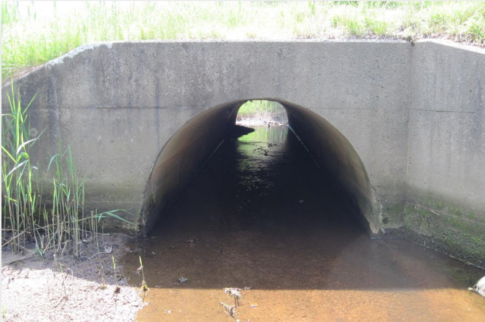
Figure 2-8. Downstream end of large Eastern Avenue culvert (culvert E).
