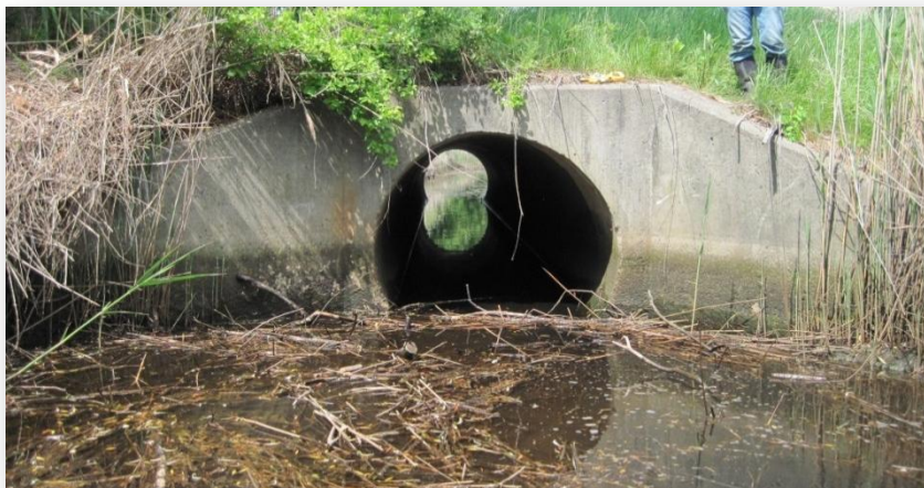
Figure 2-9. Downstream end of Gates Road Culvert (culvert D).
