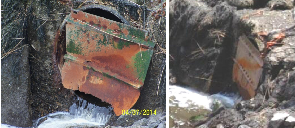
Fig. 2.20 Enlarged View of Improvised Tide Gate on North End of Ballard Street Culvert (“BA-1”)
