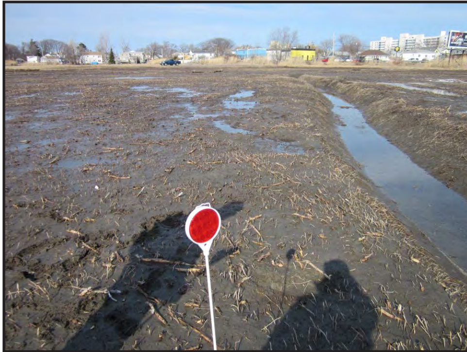
Photo F-2, Looking Northeast - March 2014.
