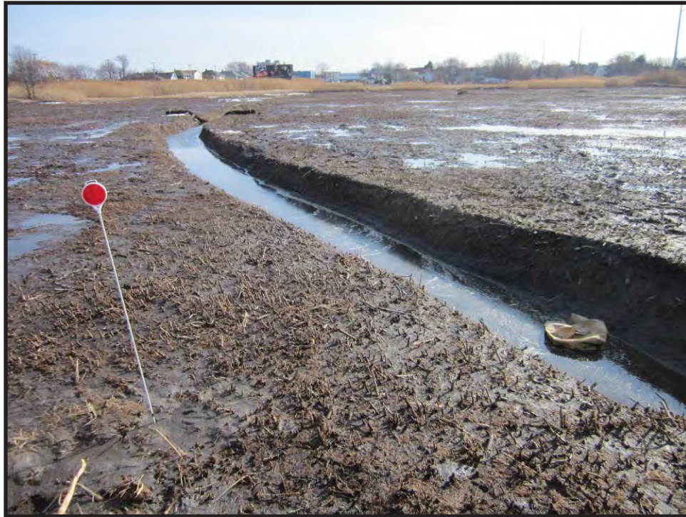
Photo B-1, Looking South - March 2014.
