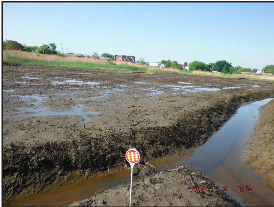
Photo E-3, Looking South - June 2014.
