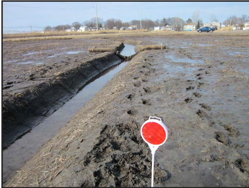
Photo E-1, Looking North - March 2014.
