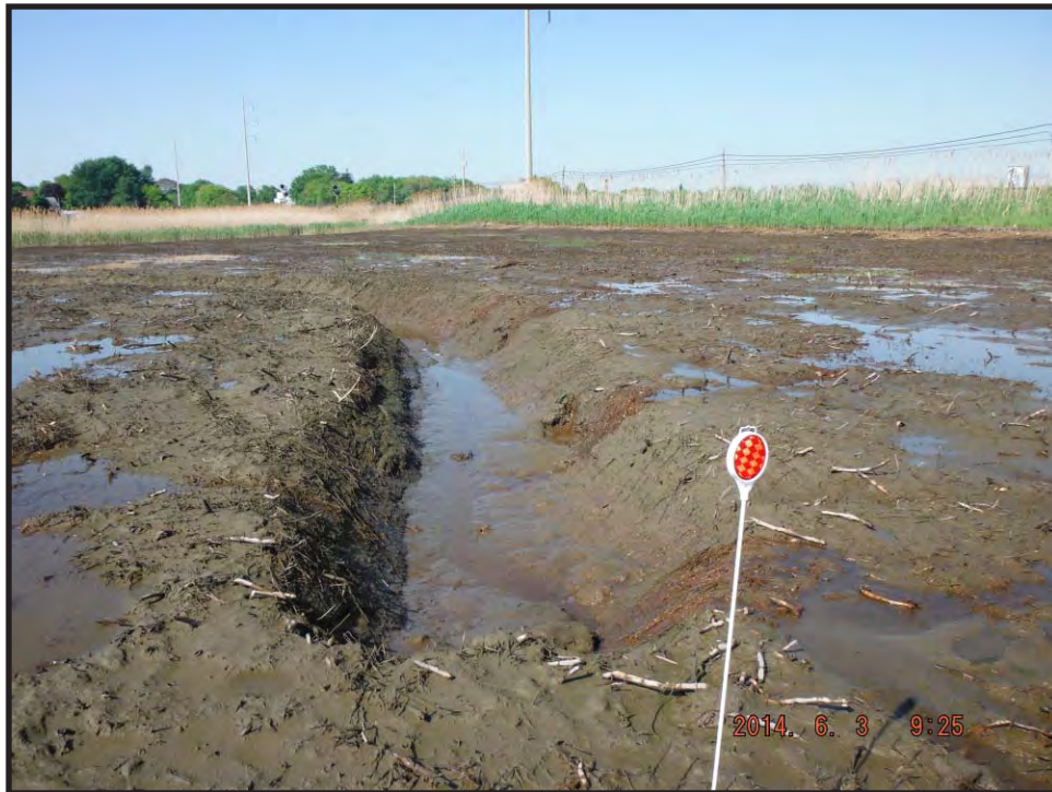
Photo G-4, Looking Southwest - June 2014.
