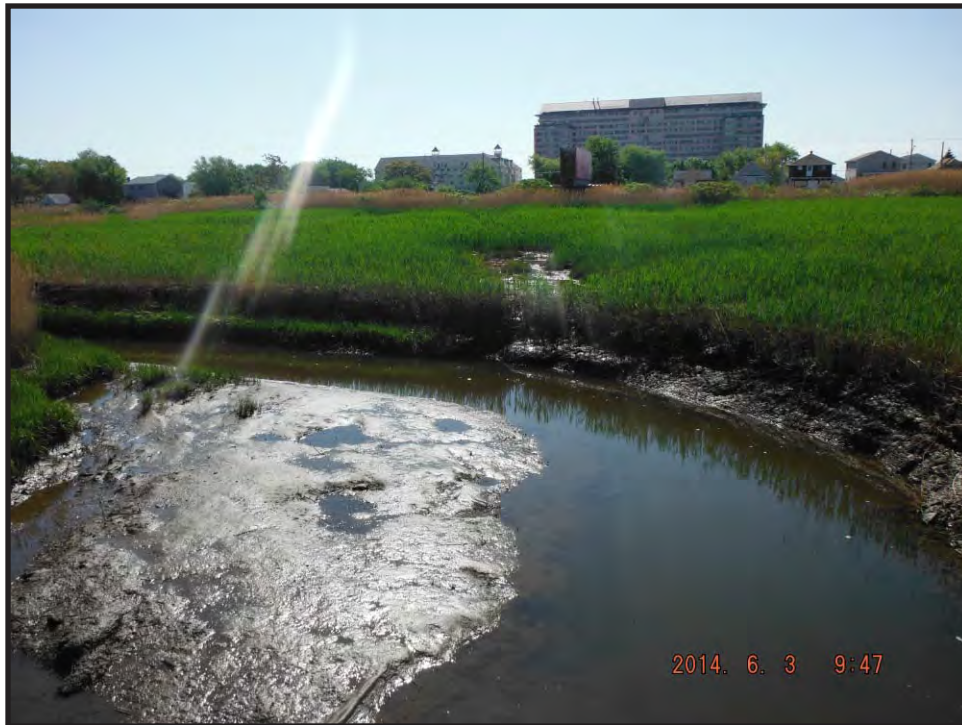
Photo Railroad Culvert 2, Looking Southeast - June 2014.
