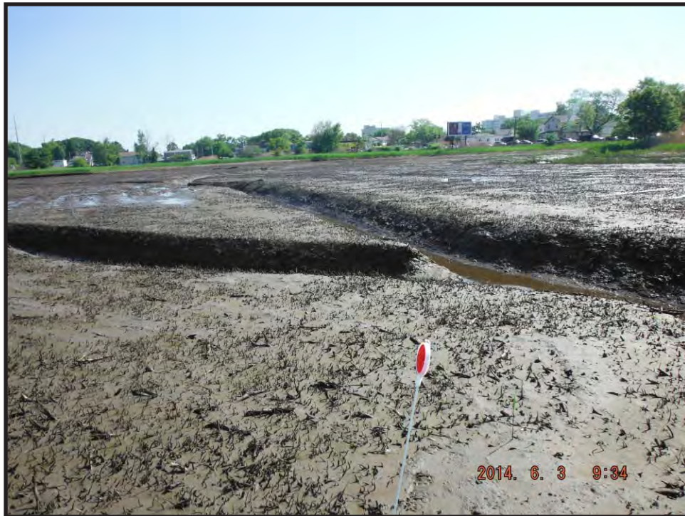
Photo K-2, Looking Northeast - June 2014.
