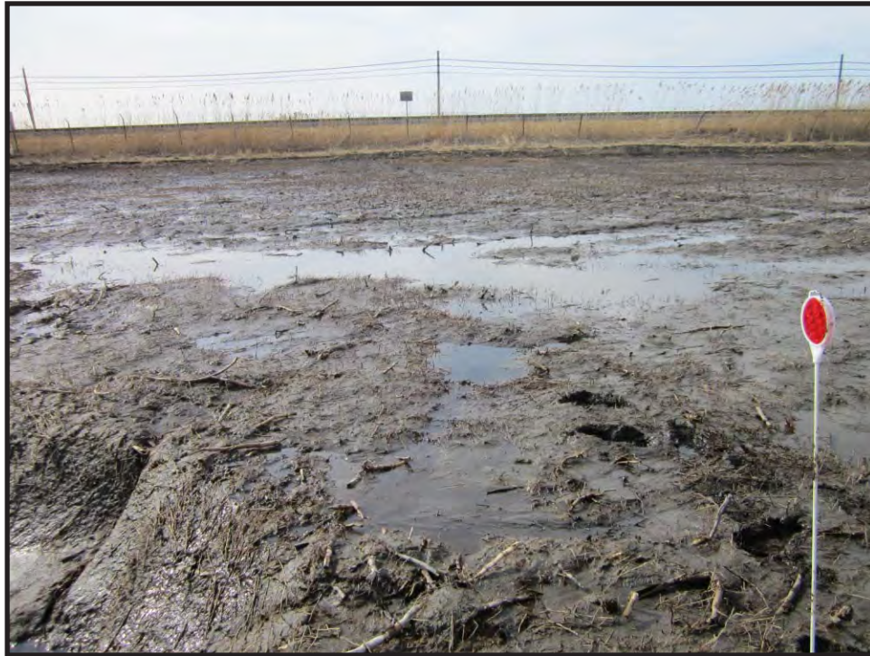
Photo G-5, Looking Northwest - March 2014.
