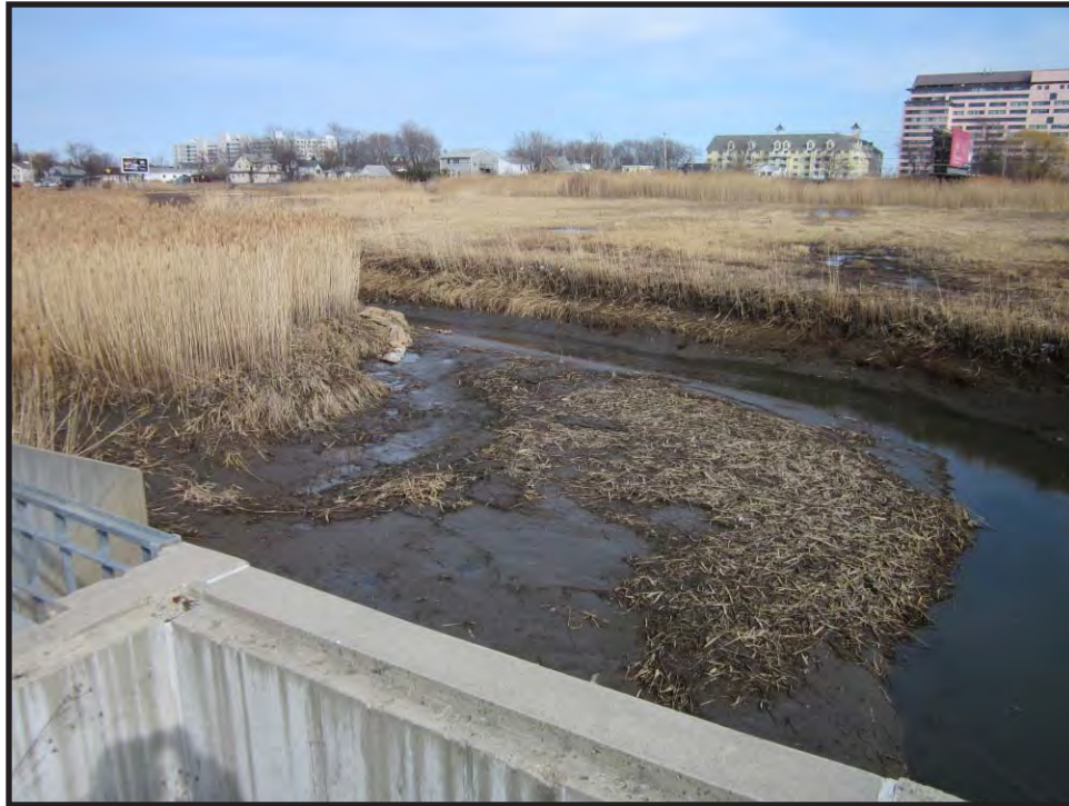
Photo Railroad Culvert 1, Looking Northeast - March 2014.
