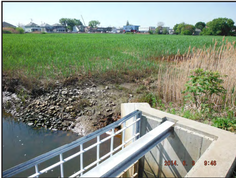
Photo Railroad Culvert 3, Looking South - June 2014.
