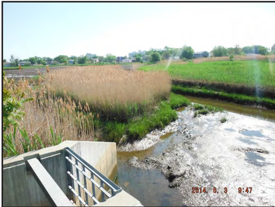
Photo Railroad Culvert 1, Looking Northeast - June 2014.
