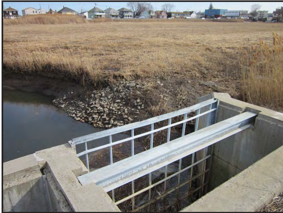
Photo Railroad Culvert 3, Looking South - March 2014.
