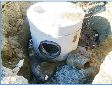
▲ Example of a drainage manhole to be installed.
