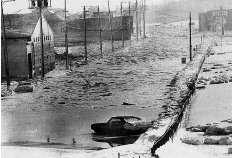
Damage from the Blizzard of 1978
