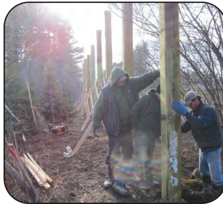
As shown above in a photo of the fence under construction, the backing rails are pressure treated 2x6s mounted to the posts using galvanized joist hangers. Below, the Main Line Fence crew plumbs the upright posts.
