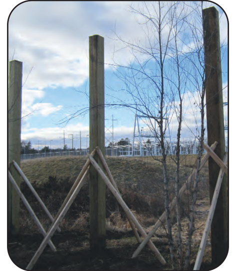
Above, uprights are braced in place while the concrete footings cure. In the background is the electrical substation from which the tall fence is designed to shield the neighborhood.
