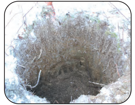
Above, one of the 24 in. wide x 48 in. deep footings, all of which had to be dug by hand.
