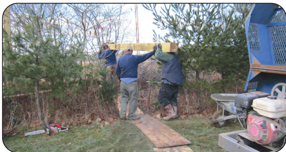
Main Line Fence crew members were required to haul all materials to the jobsite by hand, including the 12' high pressure treated uprights, weighing in the neighborhood of 350 pounds each. Other complicating factors made the installation especially difficult, including the rugged terrain, rocky and frosty soil, and winter Maine weather. Above, crew members Justin Kinne, Zane Campbell and Scott Golding hard at work.
