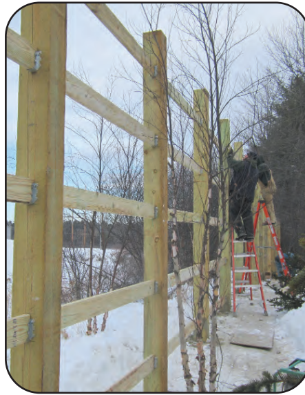
As shown above in a photo of the fence under construction, the backing rails are pressure treated 2x6s mounted to the posts using galvanized joist hangers. Below, the Main Line Fence crew plumbs the upright posts.
