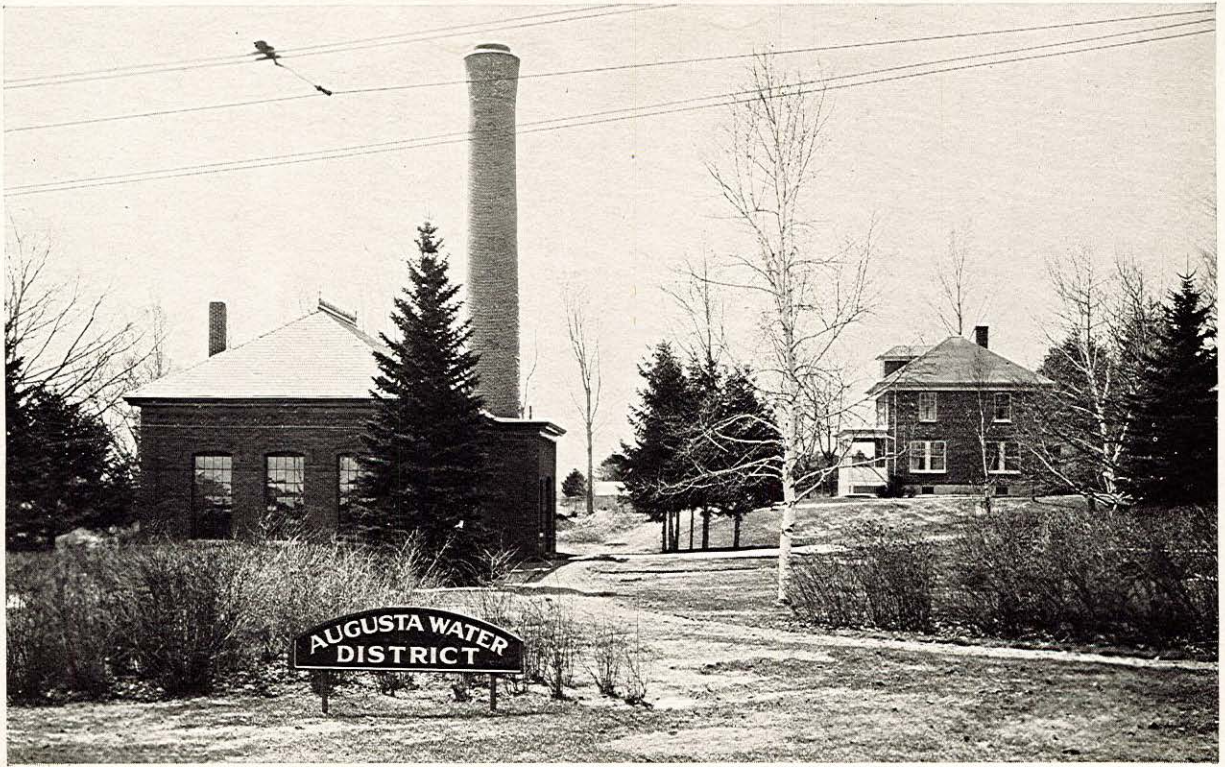
PUMPING STATION AND GROUNDS INCLUDING RESIDENCE
