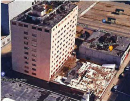
Source: Google – as seen prior to demolition.
