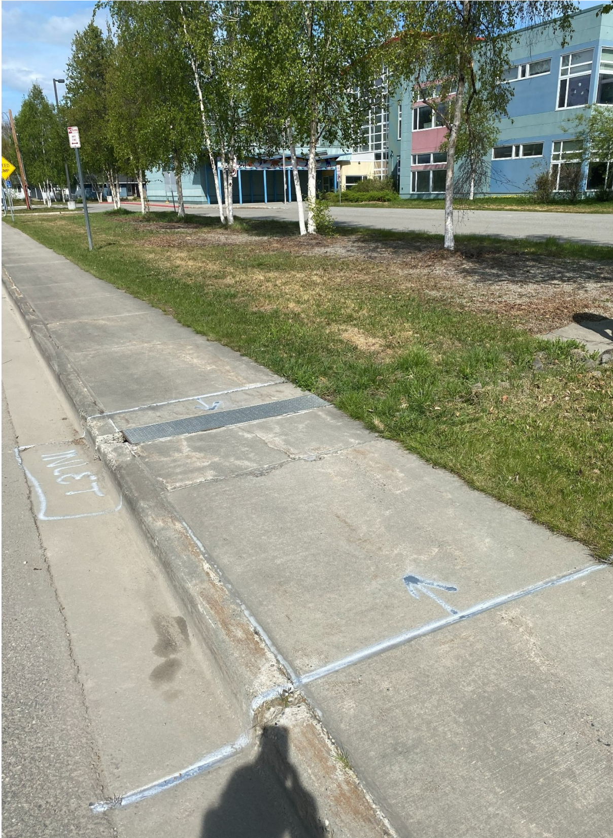
Figure 3. East side of Hamilton Street between Craig & Eureka Streets
