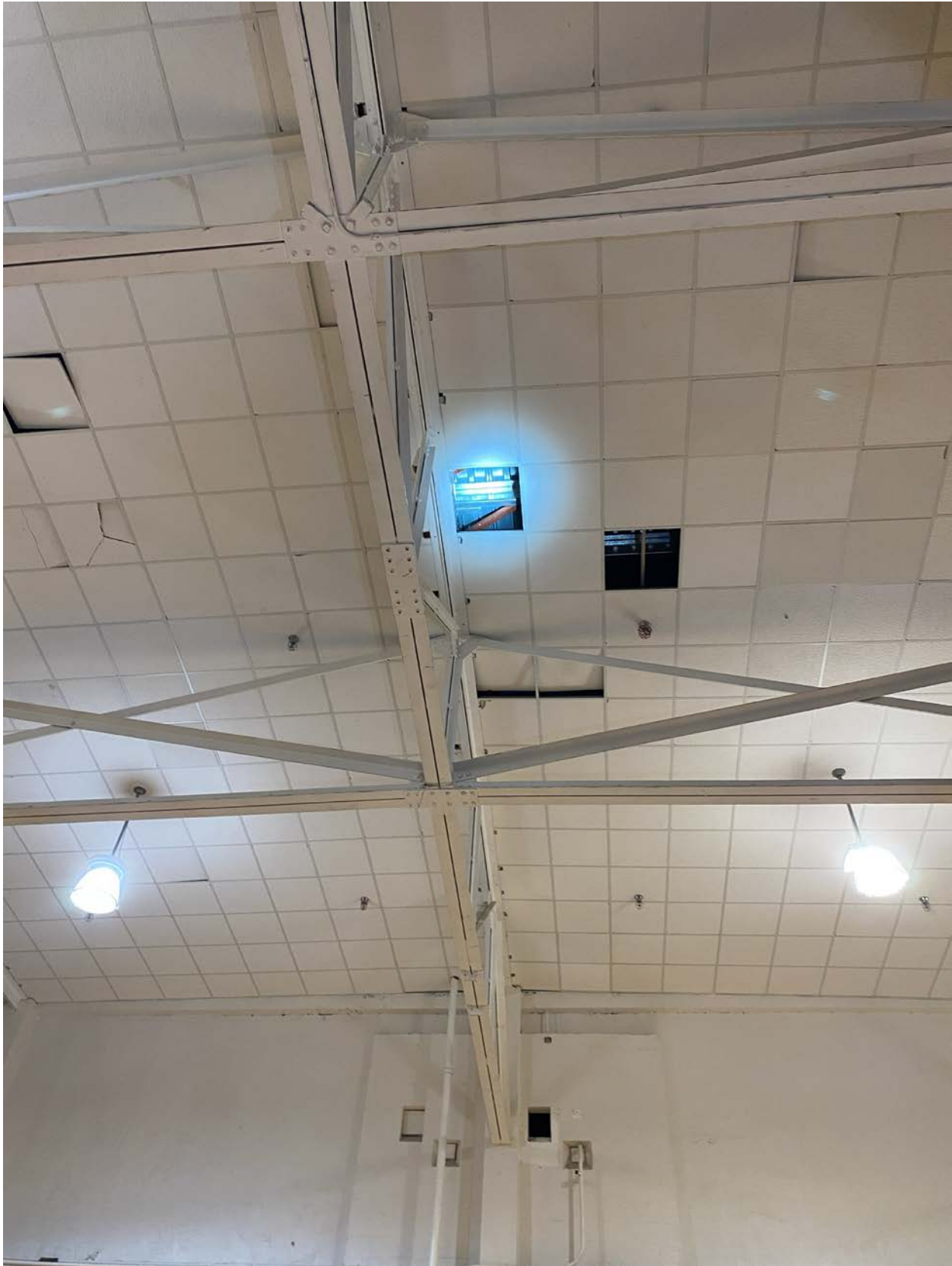
EXHIBIT 3: GYM CEILING UNDER SECTION B ROOF
