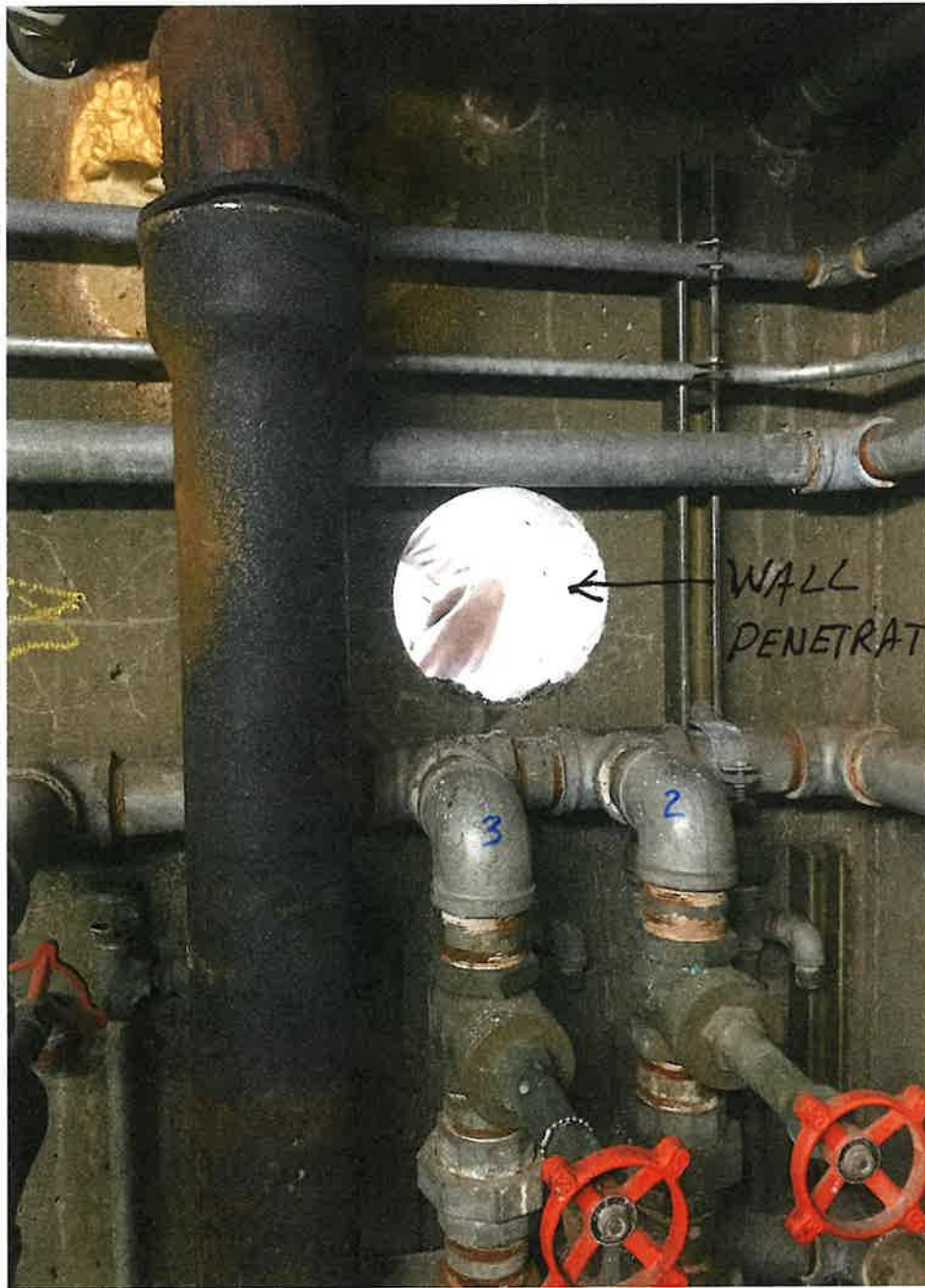
Mechanical Room → Plumbing and Penetration in Wall for 1\frac{1}{2} Ø Copper Water Service
