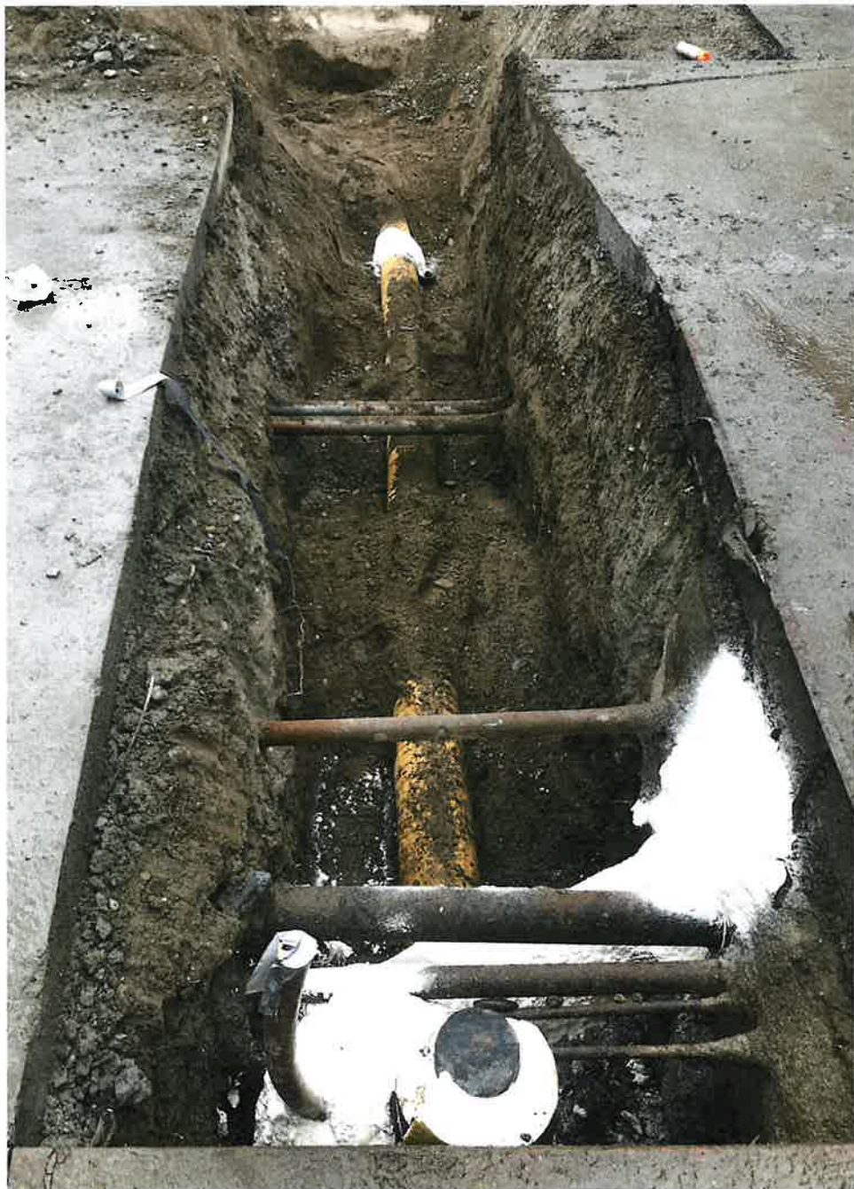
1 1/2" Copper Water Service & 4" Sanitary Sewer Service OCTOBER 2024
