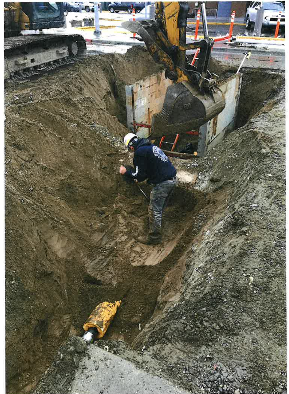
1 ST AVE. Sanitary Sewer Service Installation - October 2024
