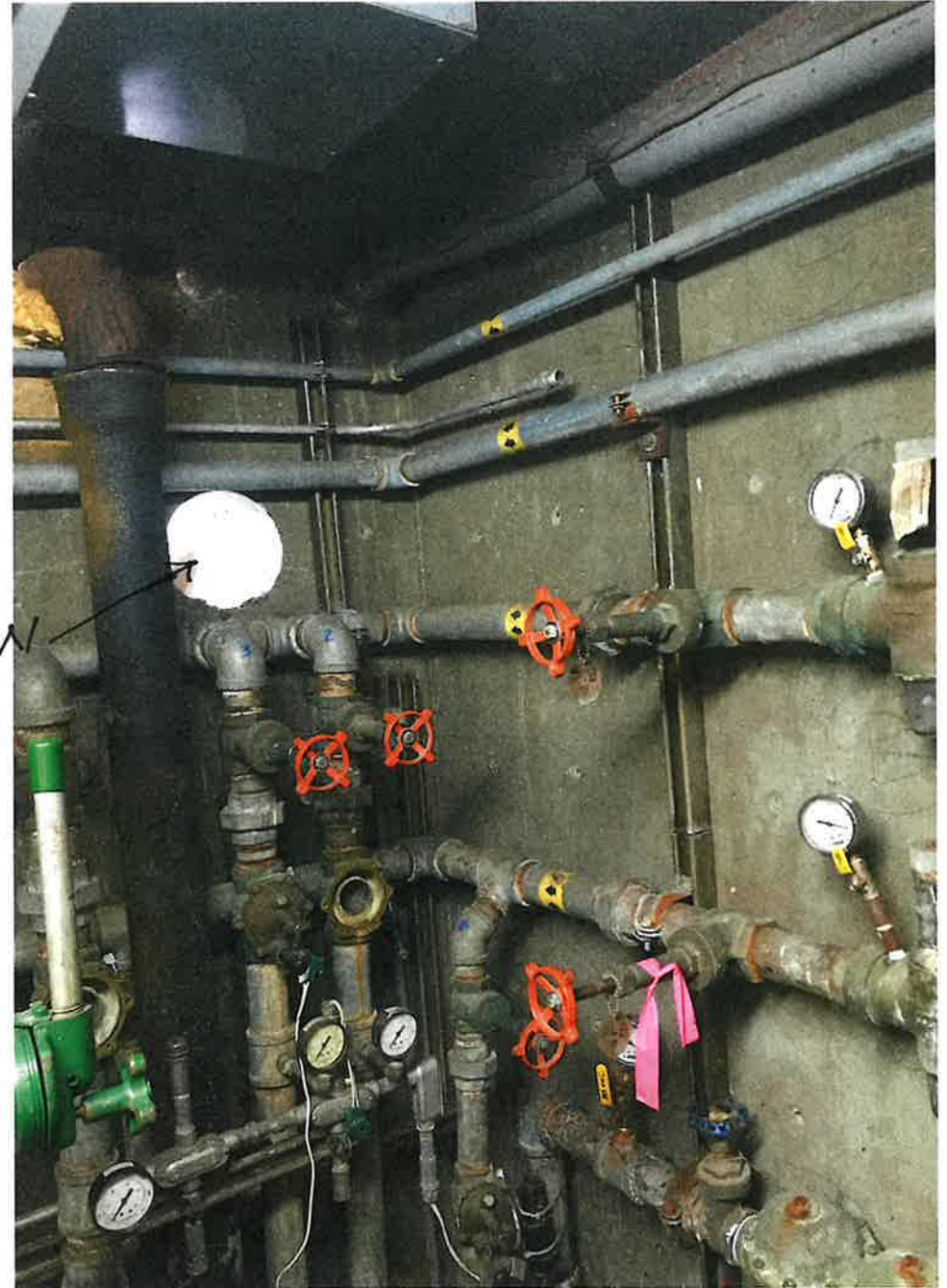
Mechanical Room → Plumbing and Penetration in Wall for 1\frac{1}{2} Ø Copper Water Service
