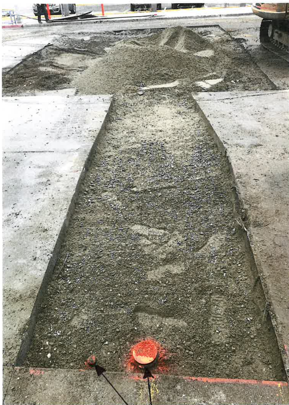
1 1/2" Water Service → 4" Sanitary Sewer Service
