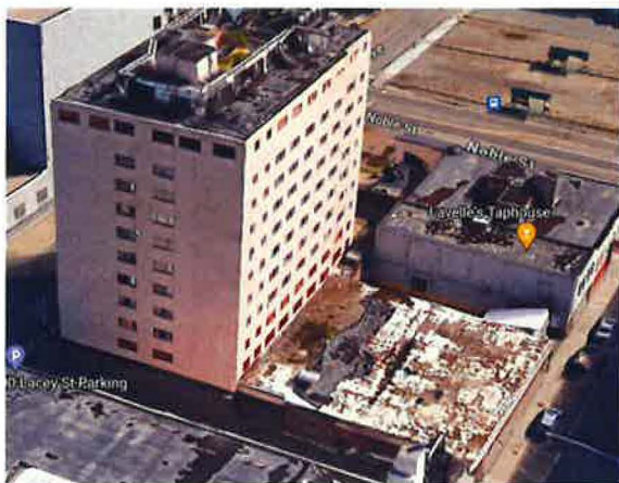
Source: Google – as seen prior to demolition.
