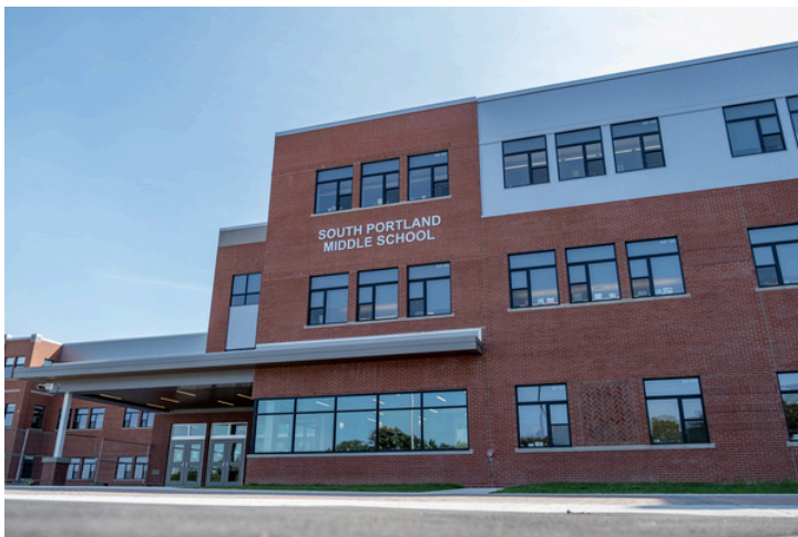
South Portland Middle School Exterior
