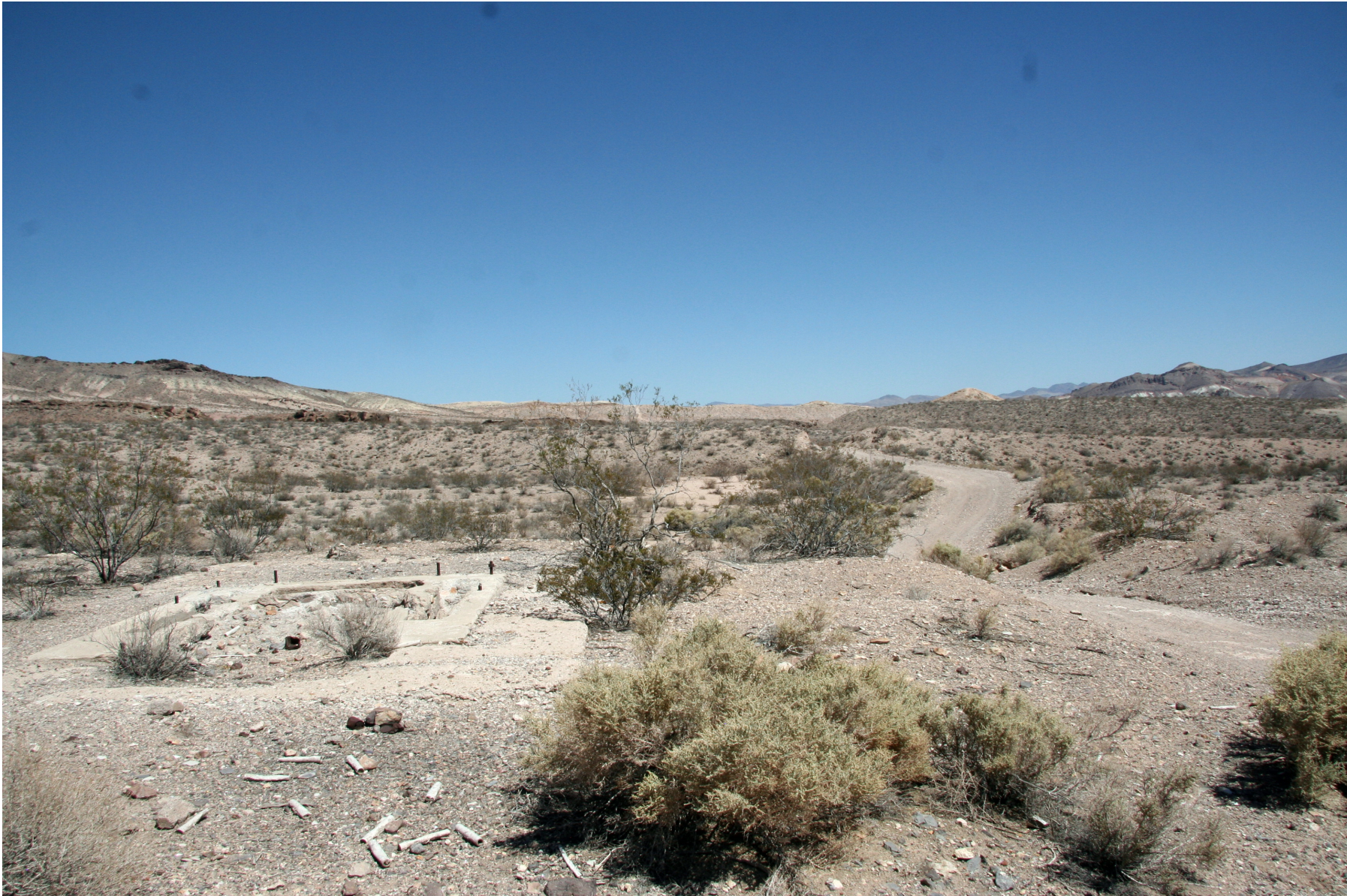
Water Lifting Station, taken by Bob Adams, September 16, 2014
