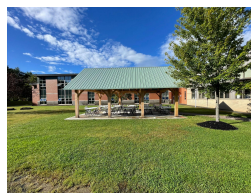
The formerly constructed MBC Pavilion
